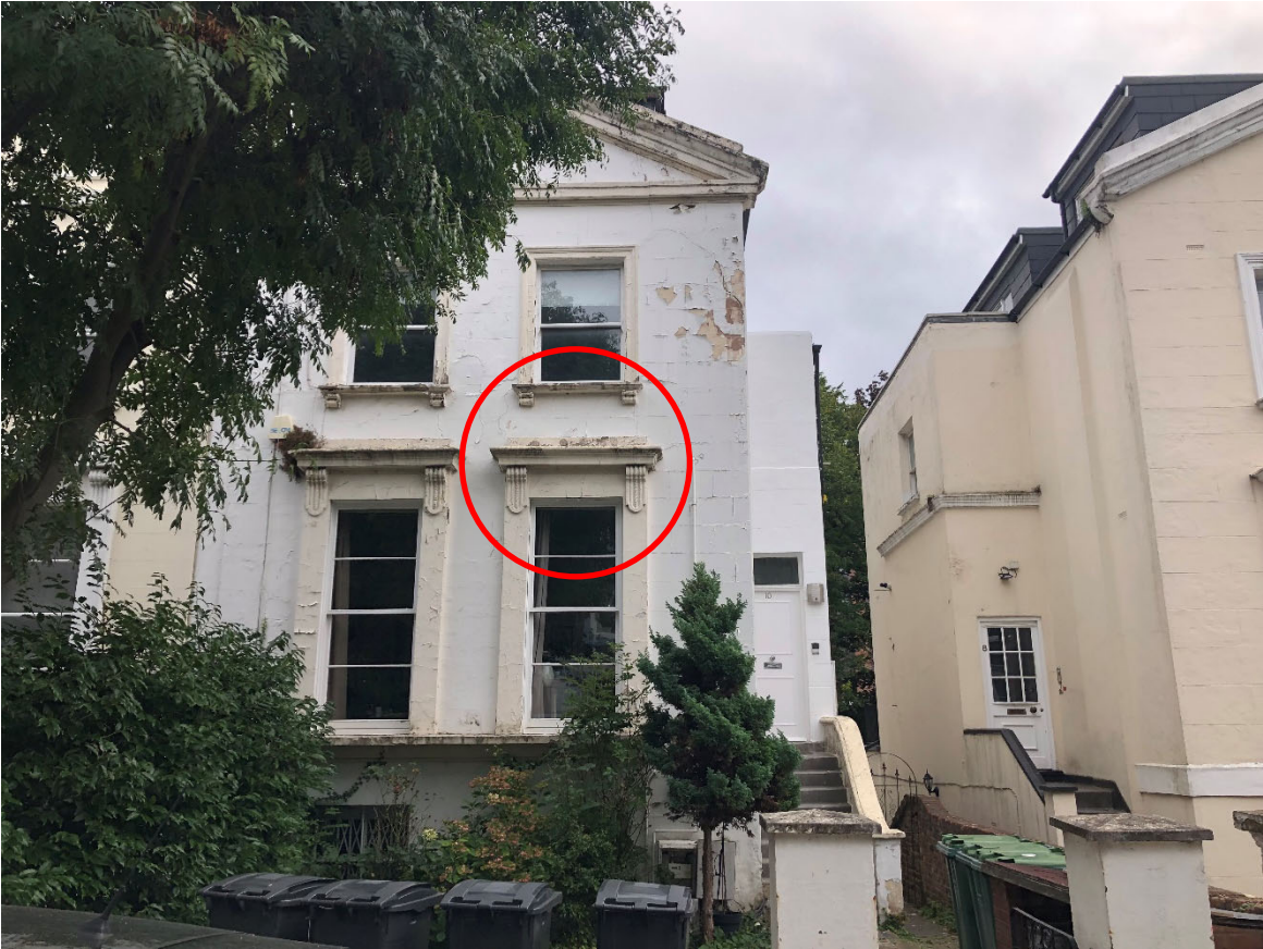
Projecting cornice over upper ground windows.
