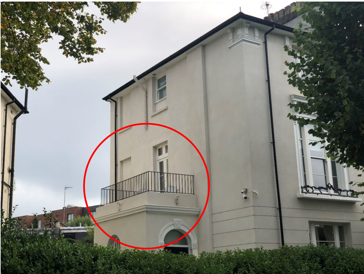
Simple black painted metal railings above entrance door.
