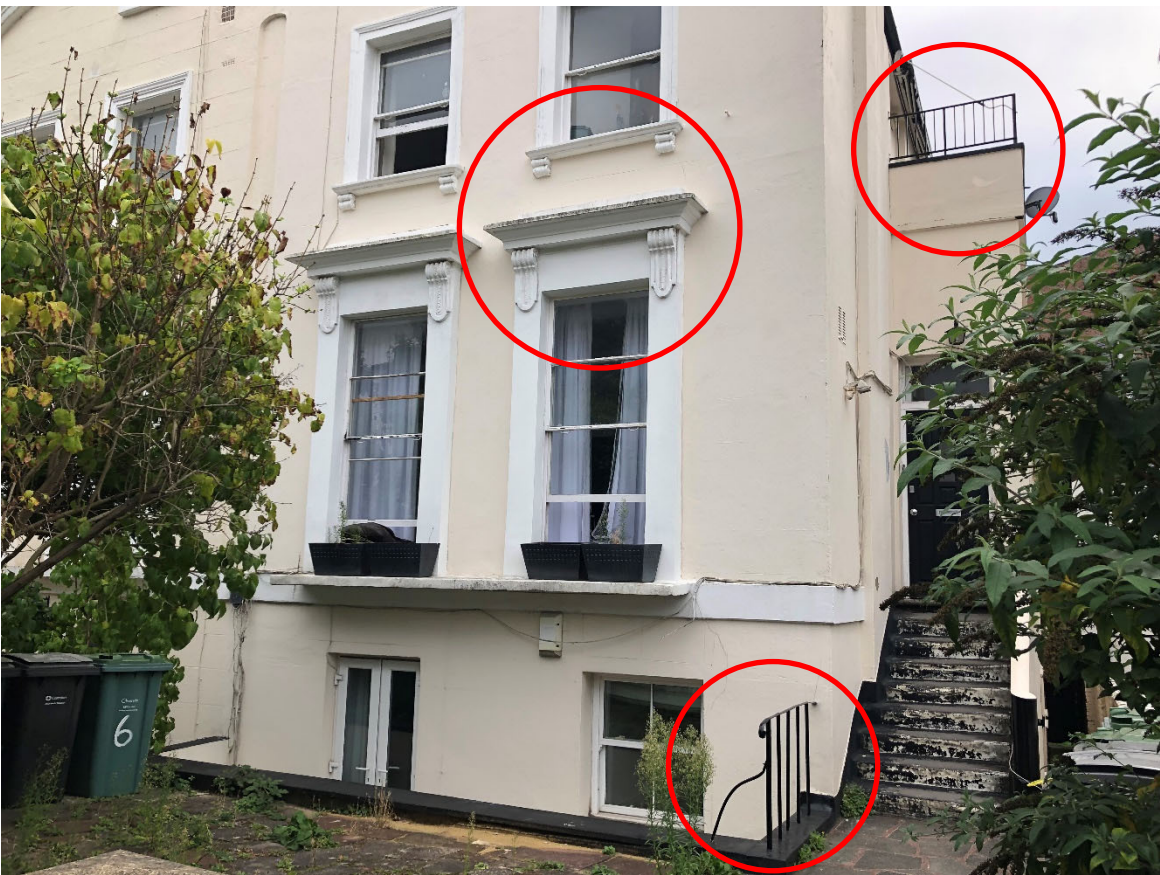
Projecting cornice over upper ground windows and simple black painted metal railings.
