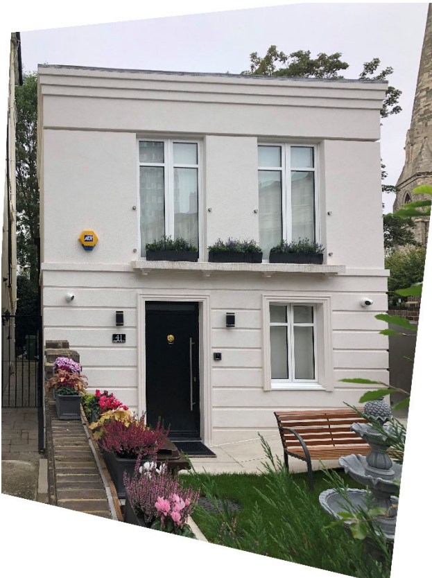
Photo of existing front façade.
