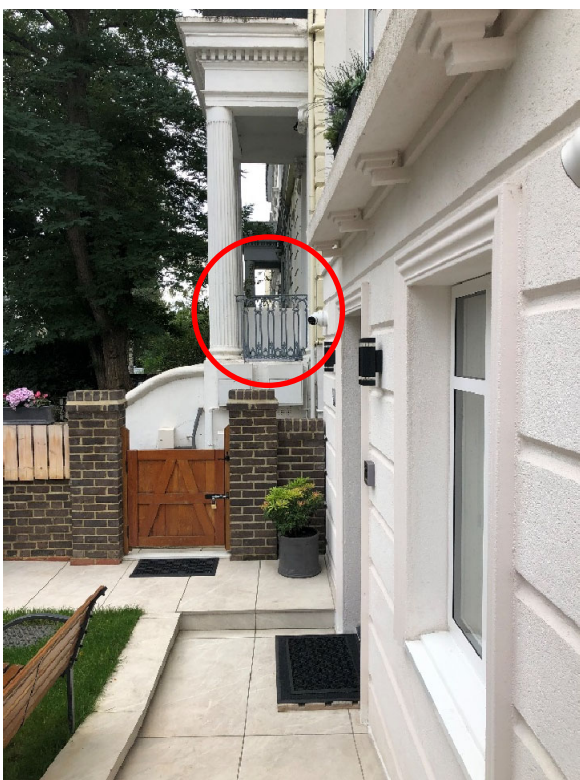
Black painted guarding at upper ground level.
