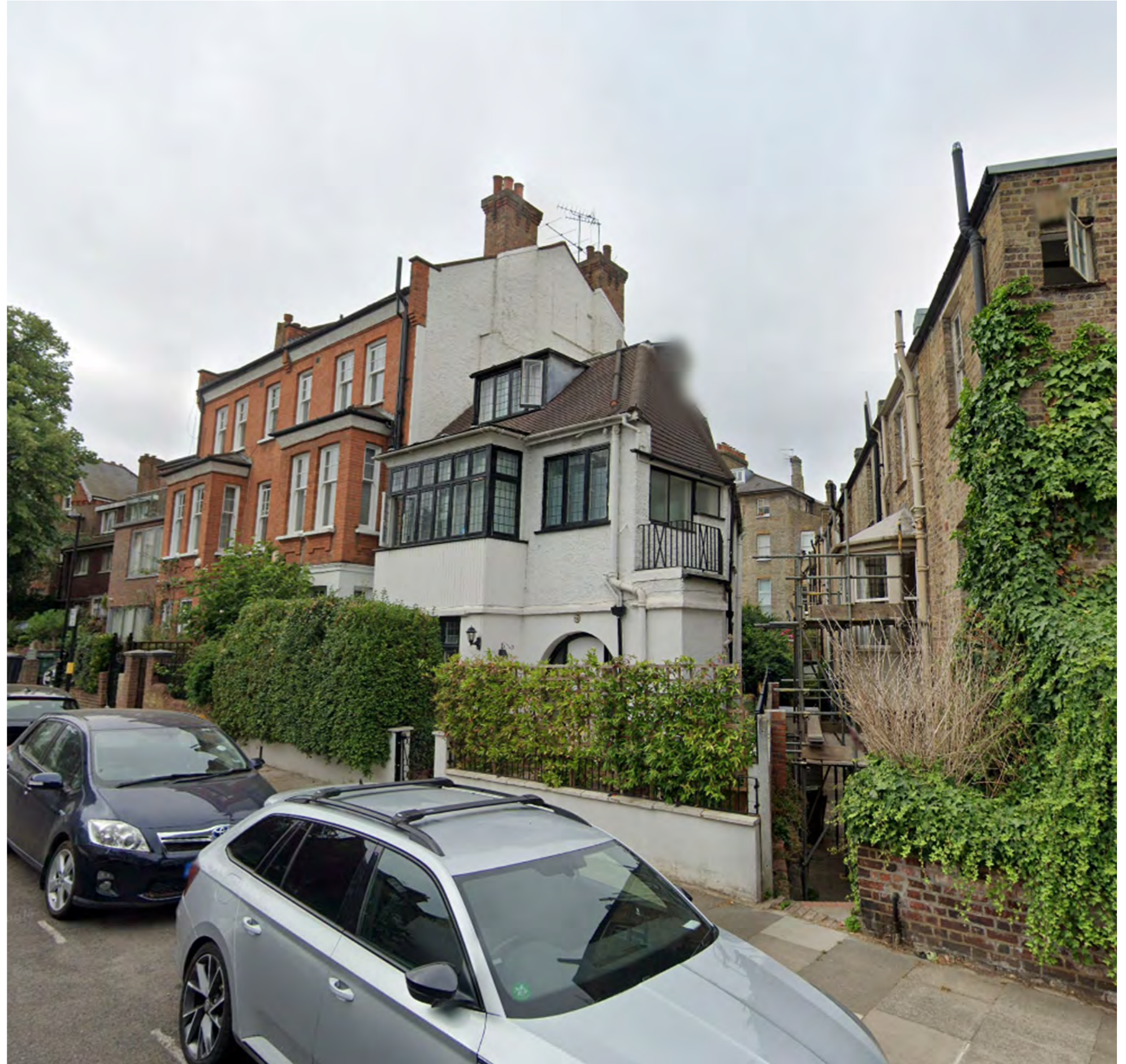
Fig. 8 - 33 WR to centre, Willow Cottages to the right, 31 WR to the left
