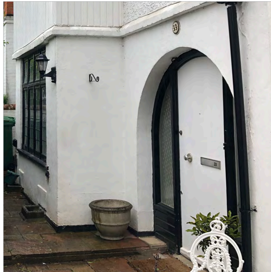
Fig. 18 - Existing sidelights with solid low-level panels
