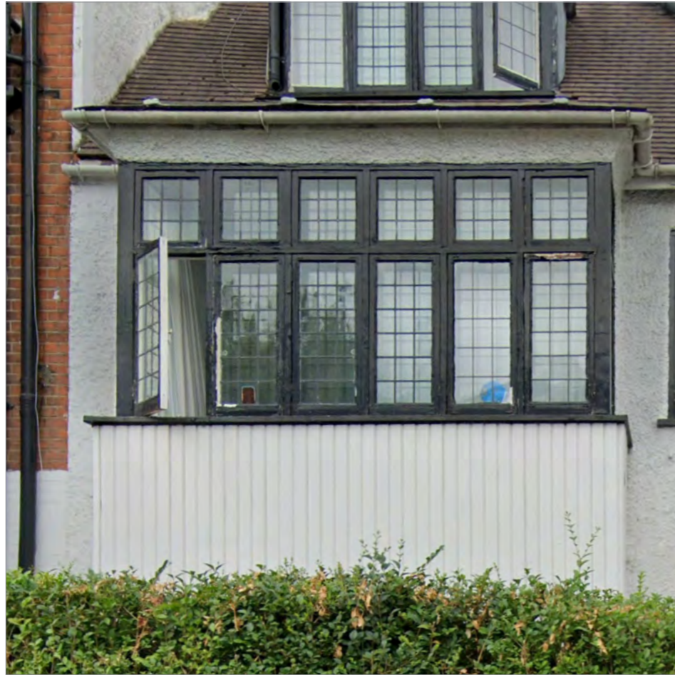
Fig. 11 - Existing First Floor Bay
