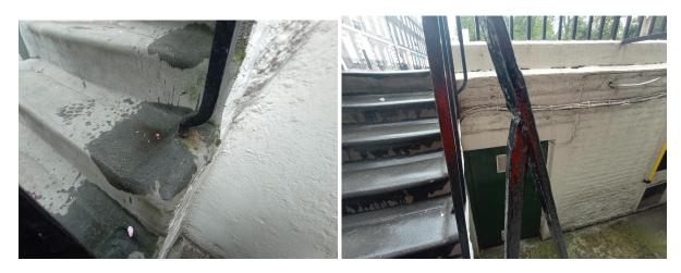
The bottom of the baluster has rusted through and is drawn so the bottom is offset from the main baluster. The top of the baluster is chamfered and appears to be riveted to the handrail. The baluster is a simple square section.
