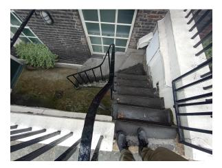
General overview of the railings at No 2 Bedford Square. The railings provide guarding to the front lightwell area. There are also railings and balustradings guarding the outer edge of the winder steps leading to the basement of the building.
