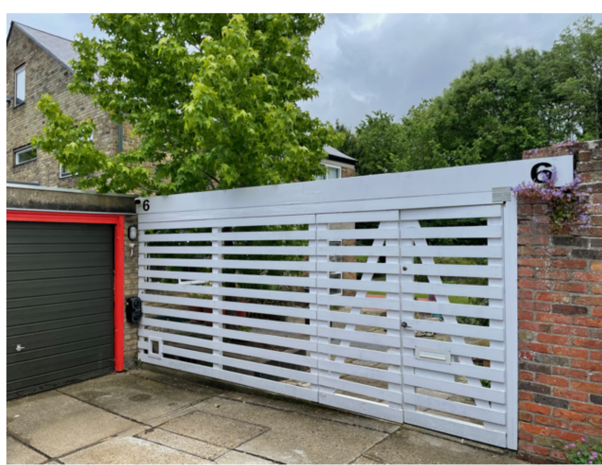
PHOTO 1: EXISTING TIMBER GATE NOT TO SCALE
