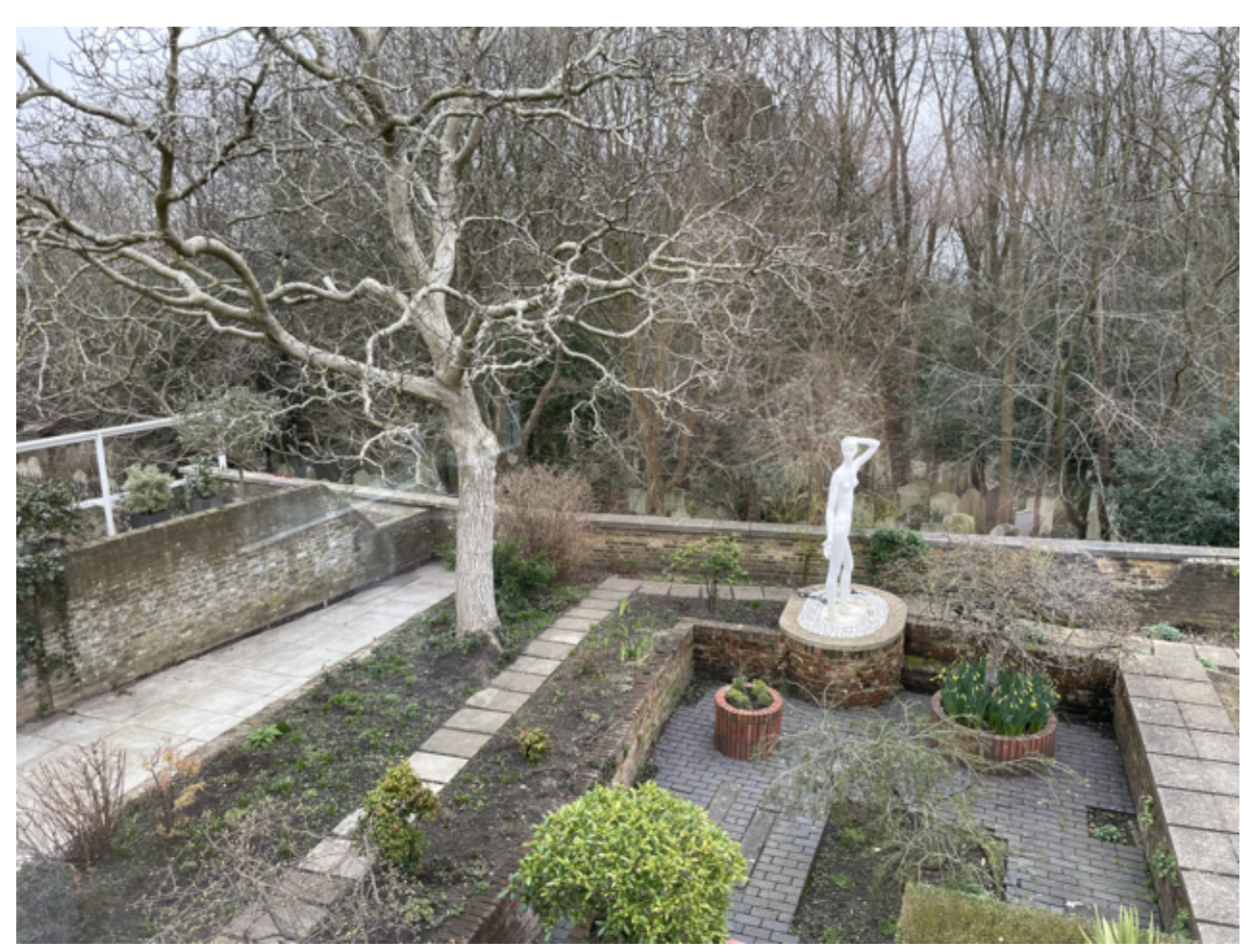
PHOTO 2: REAR WALL TO HIGHGATE CEMETERY LOOKING SOUTH EAST FROM FIRST FLOOR OF HOUSE NOT TO SCALE
