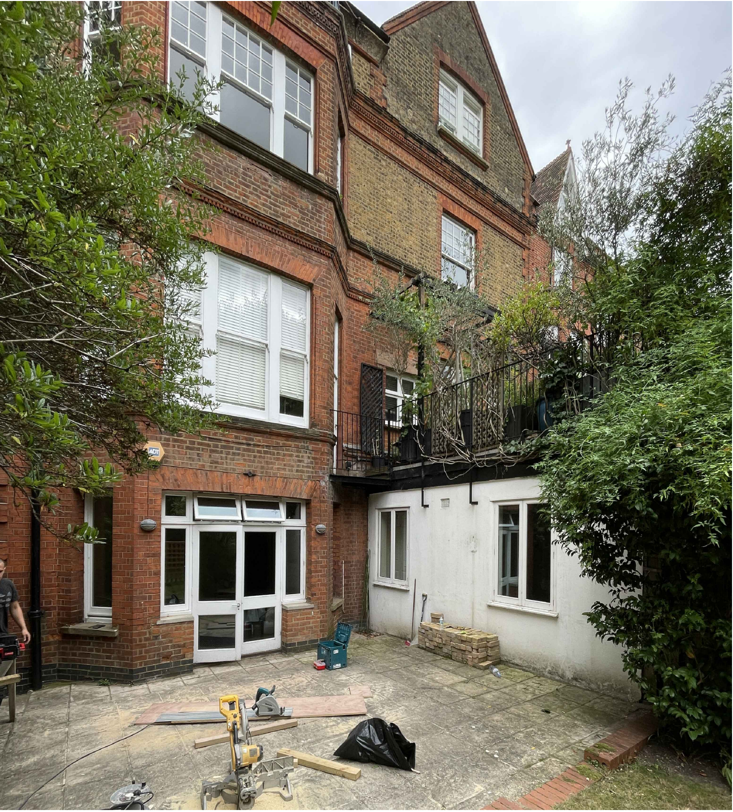
PHOTO OF EXISTING
