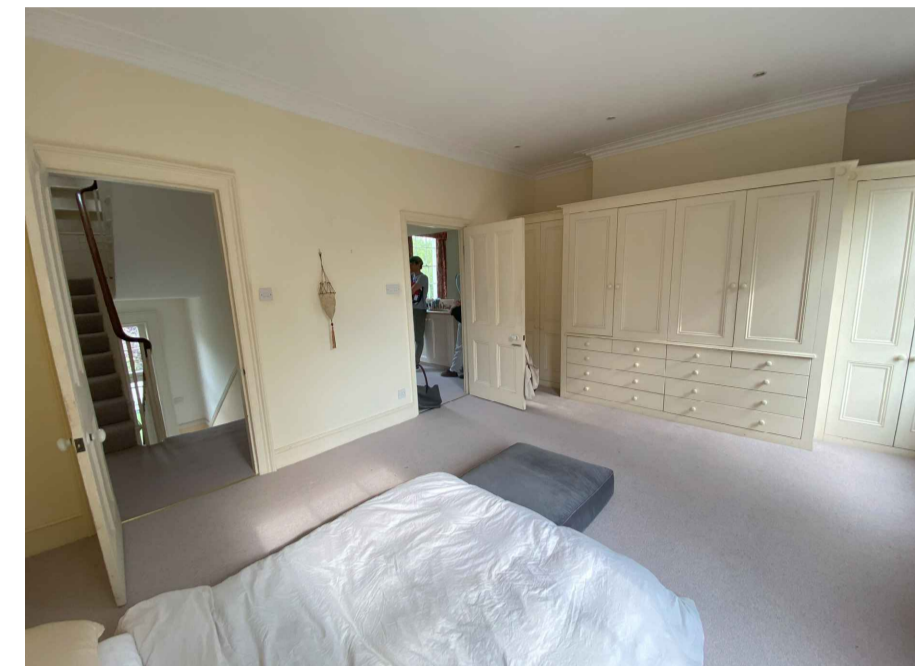
6 Master Bedroom - Joinery To Be Stripped image SCALE 1: na
