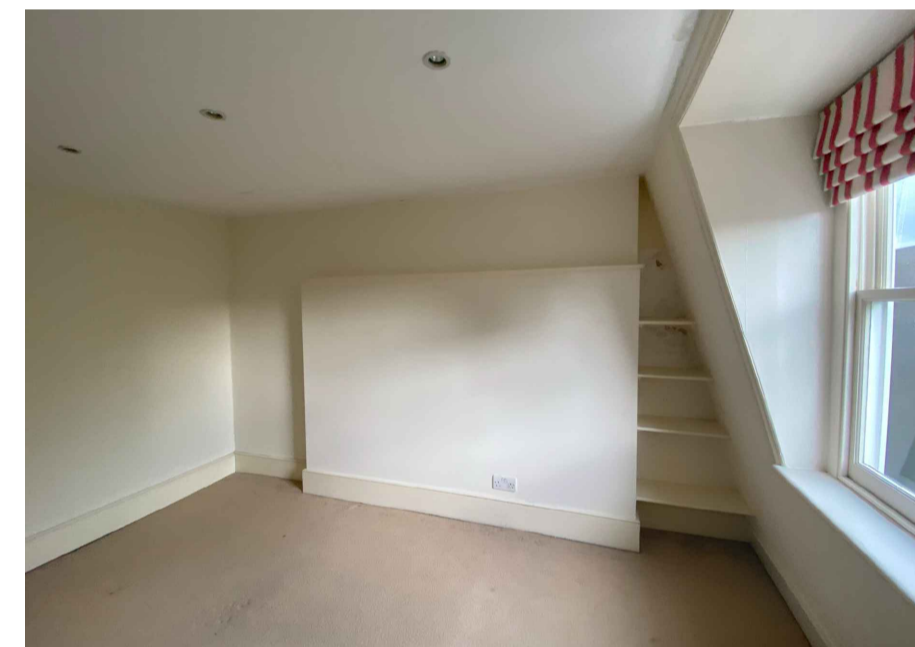
10 Third Floor Front Bedroom - Downlights To Be Removed image SCALE 1: na
