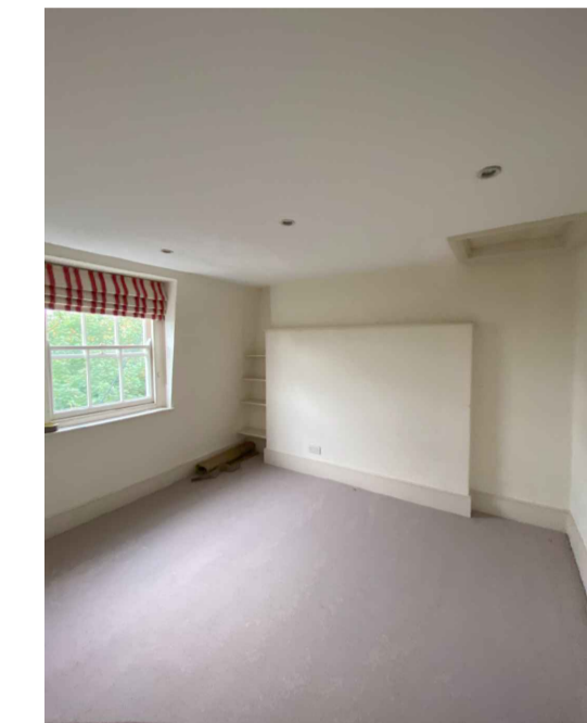
9 Third Floor Rear Bedroom - Damage To Ceiling image SCALE 1: na
