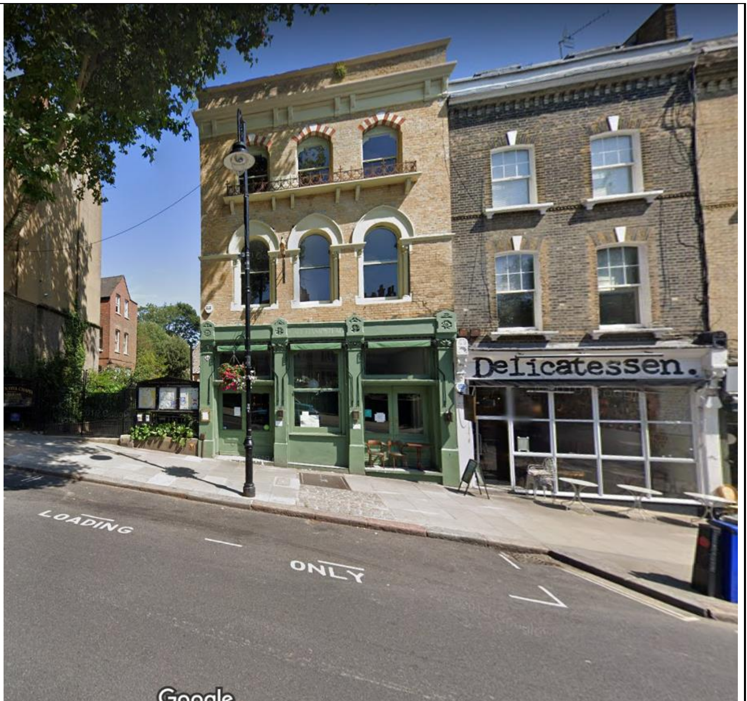
Figure 2: Pre-existing shopfront (Google Streetview July 2019)
