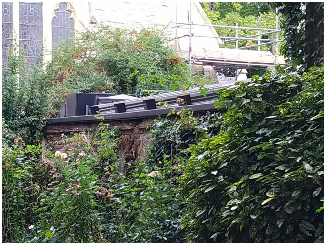
Figure 10: As built view from church yard
