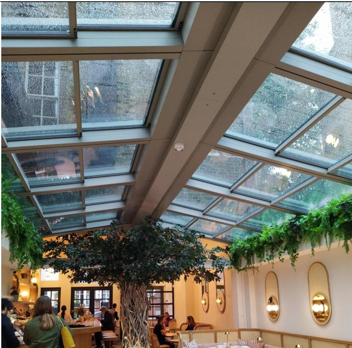
Figure 11: As built view from inside the premises
