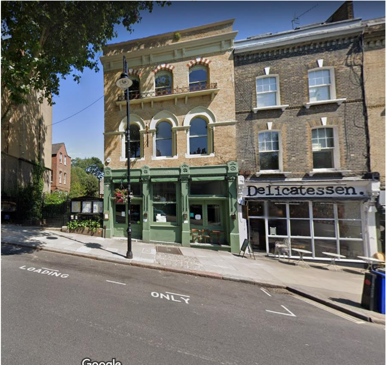
Figure 2: Pre-existing shopfront (Google Streetview July 2019)
