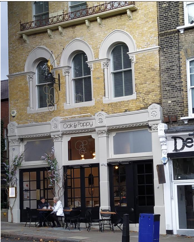
Figure 12: Shopfront with 2 x heat lamps
