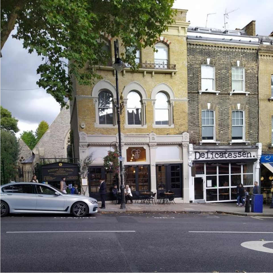
Figure 1: Site photograph showing the existing front elevation of the restaurant
