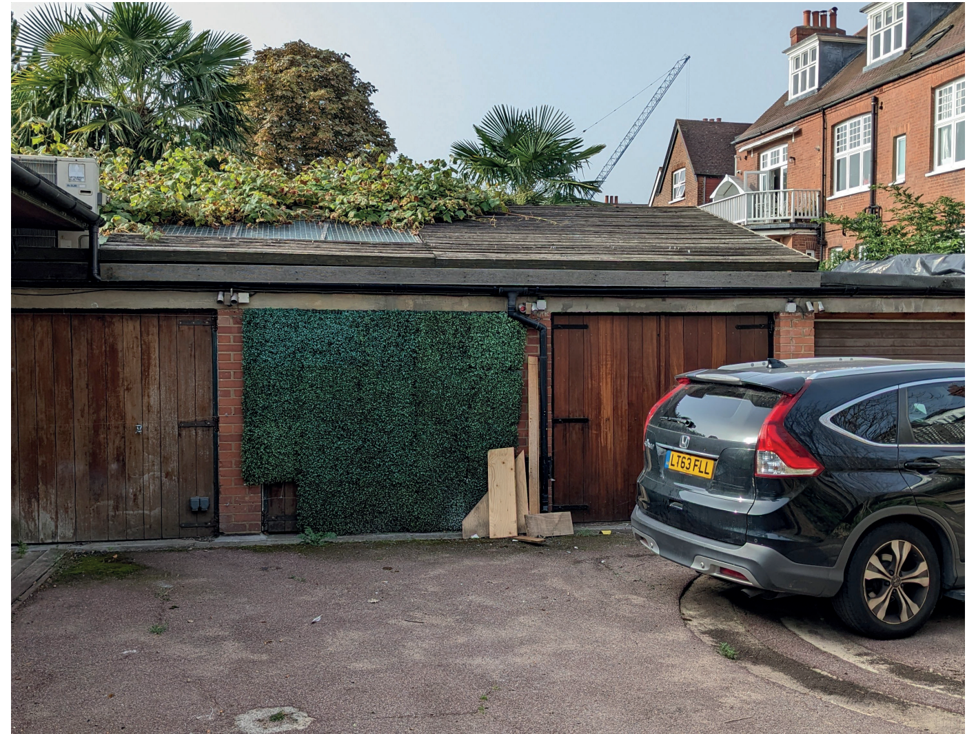
Existing Garage Buildings
