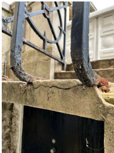
Stair 03: Original stone stair faced with failing cementitious render, very thin original cantilevered landing
