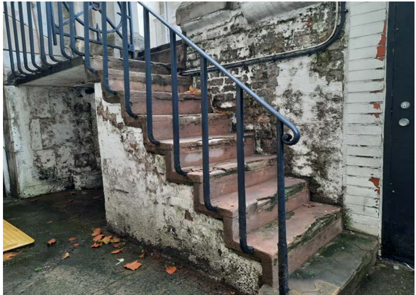
Stair 03: Original stone stair faced with failing cementitious render, very thin original cantilevered landing
