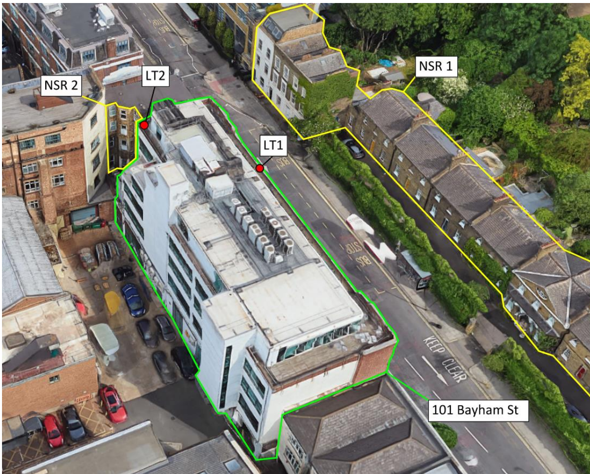
Figure 2: Location of long-term survey, and locations of existing sources of plant noise at the site.
