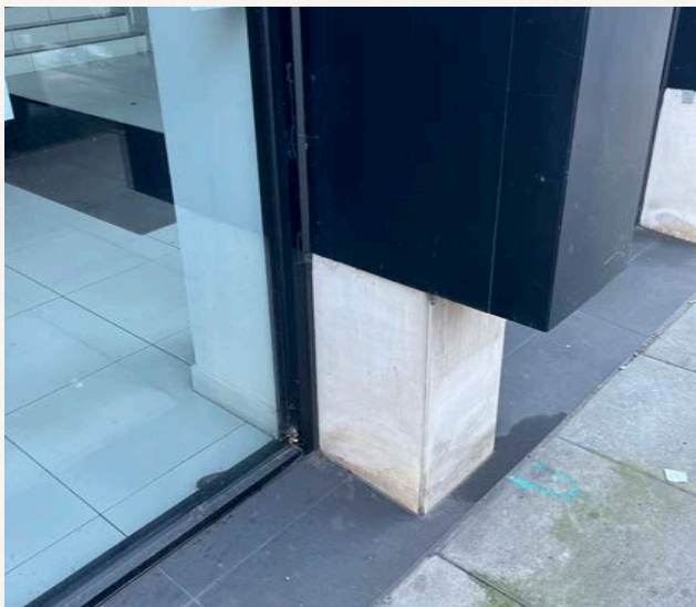
Metal fascia removed stone pier exposed beneath
