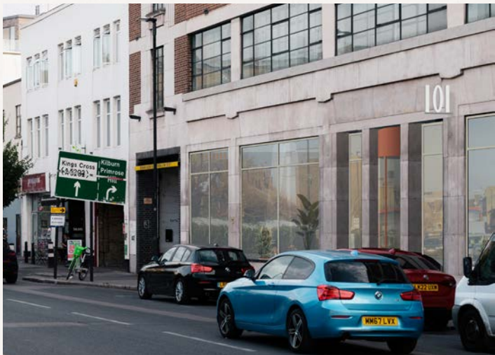
The elevation is enlivened by removing window film. Recently added steel cladding is removed to expose the existing underlying stone piers.
