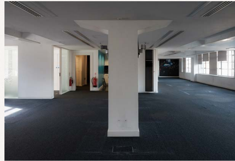
The existing structure and character of the interiors has been overclad in plasterboard.
