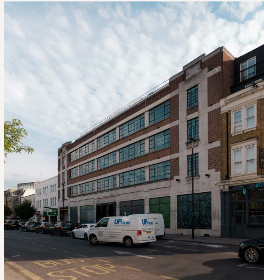
Railpen own the site at 101 Bayham Street
