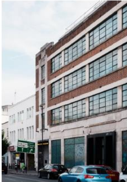
101 Bayham Street, existing external view
