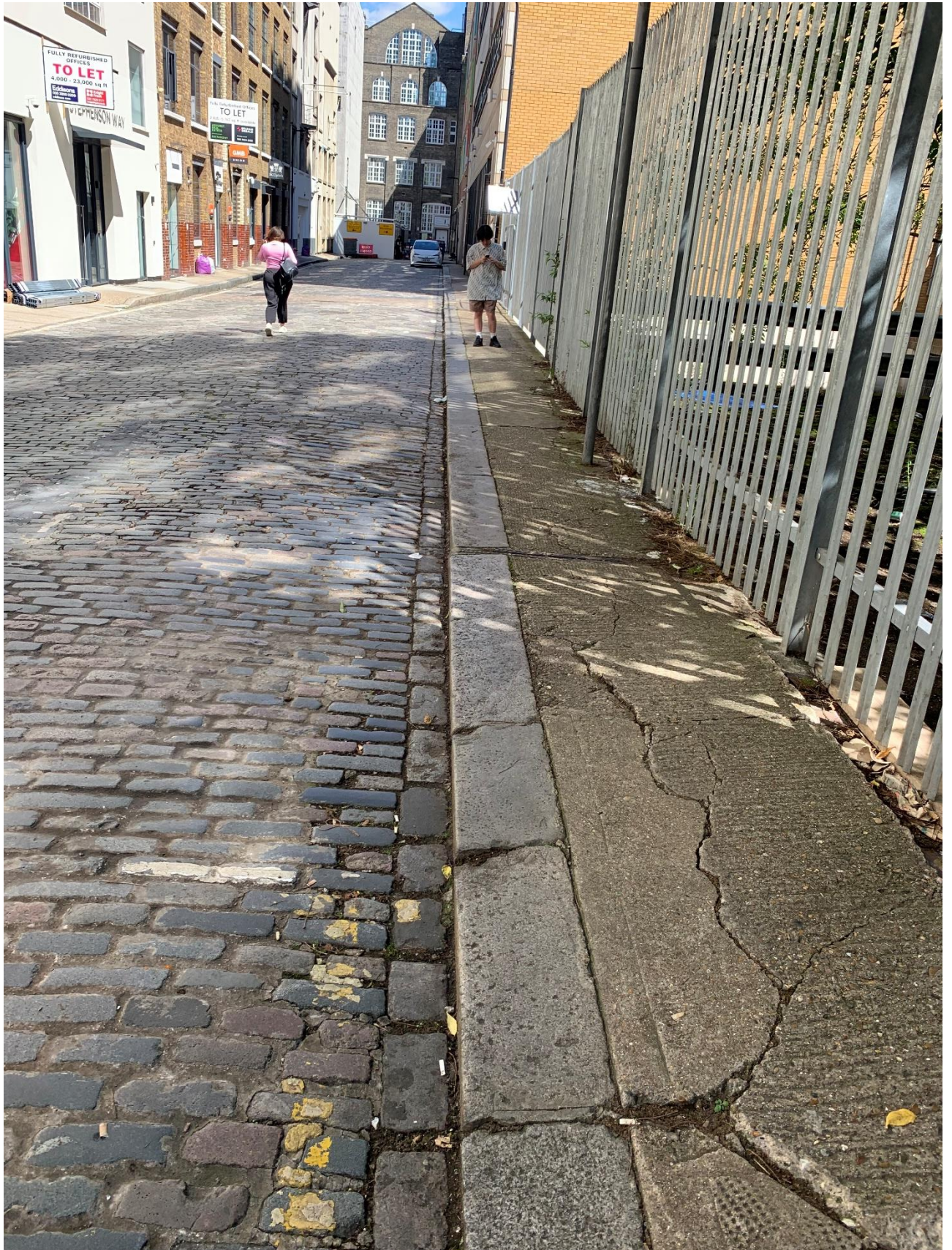
Photo 1: The granite setts in their present condition.
