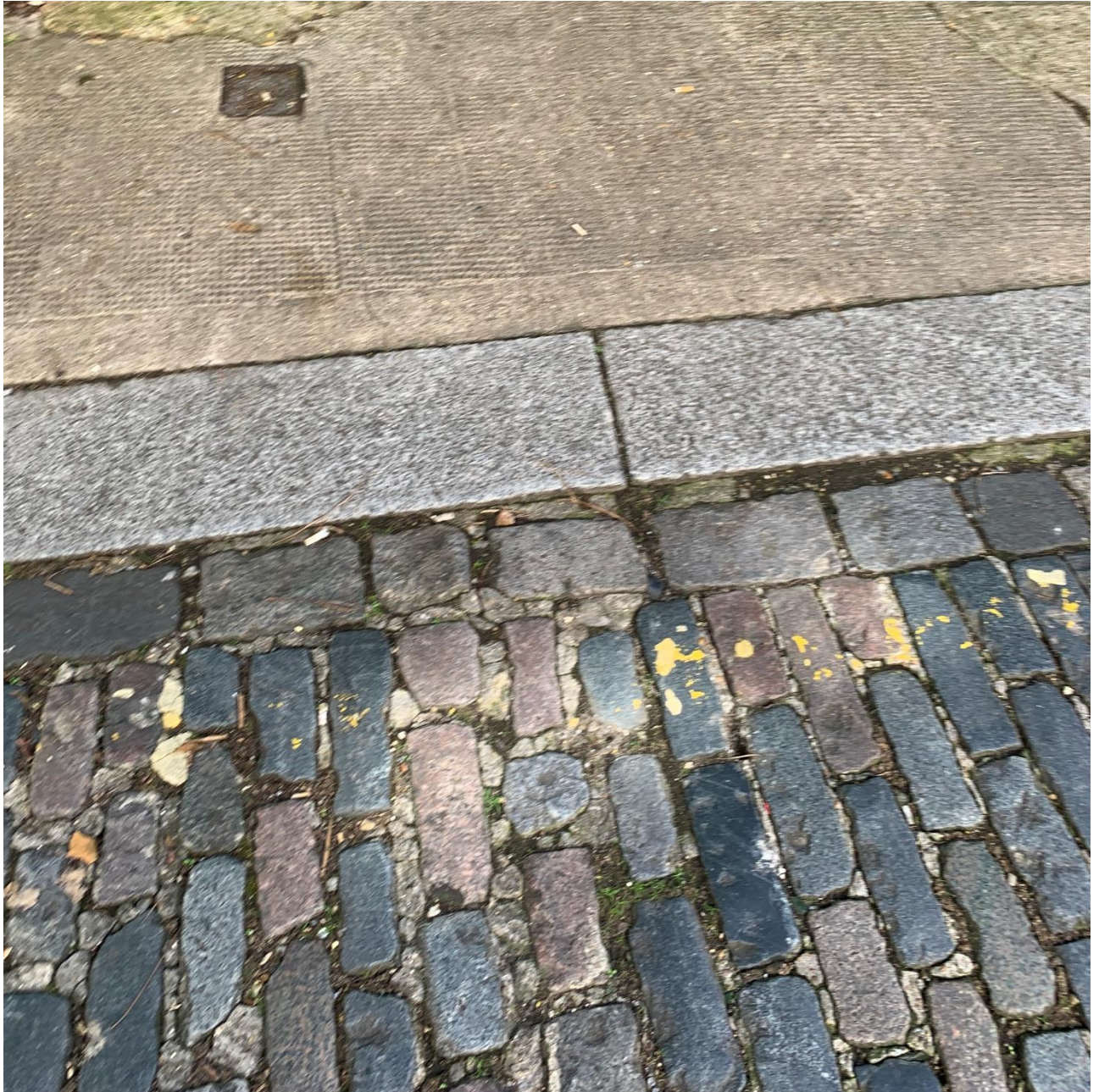
Photo 4: A detailed photo, showing the present condition of the granite setts and dropped granite kerb.
