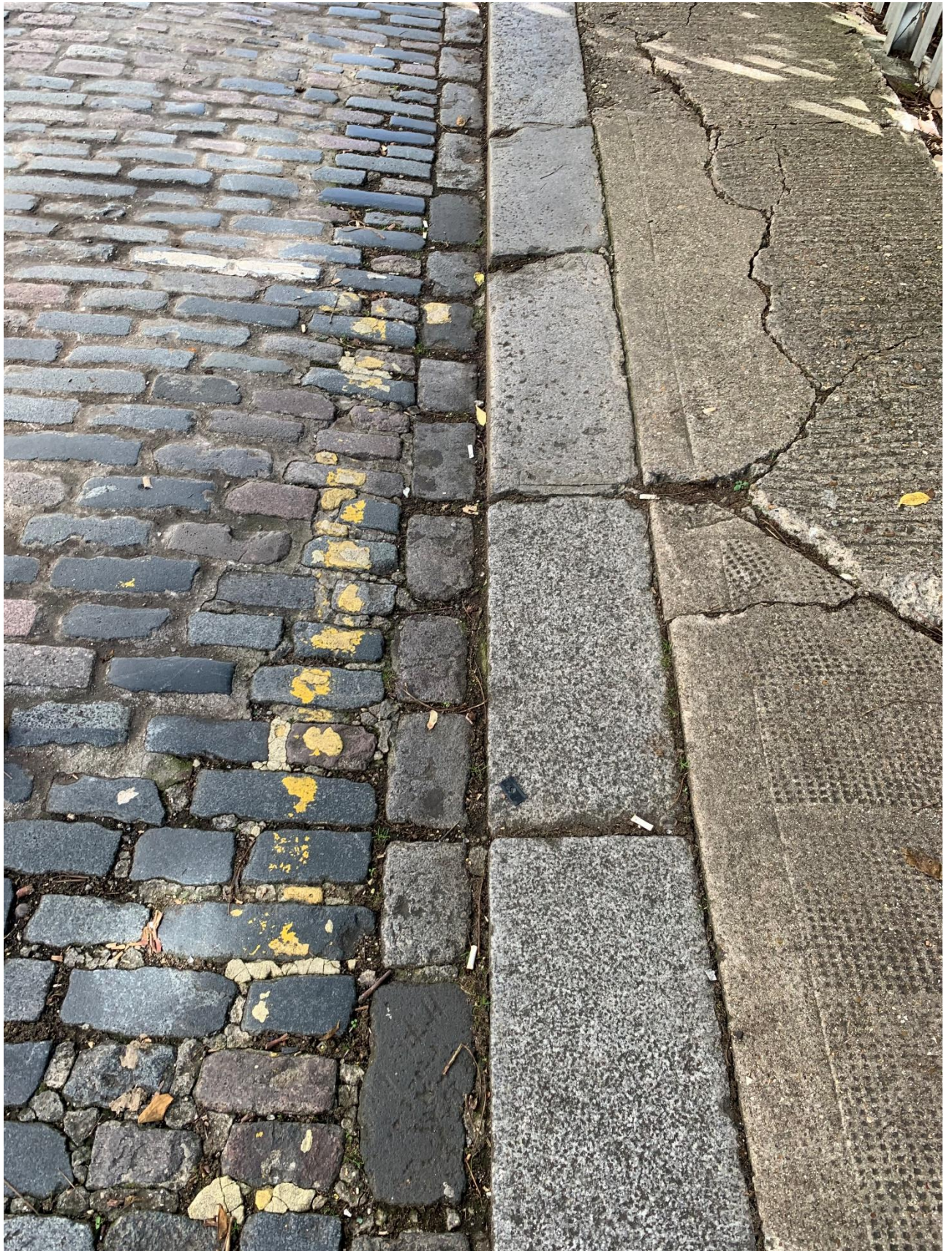
Photo 2: A detailed photo, showing the present condition of the granite setts and granite kerb.
