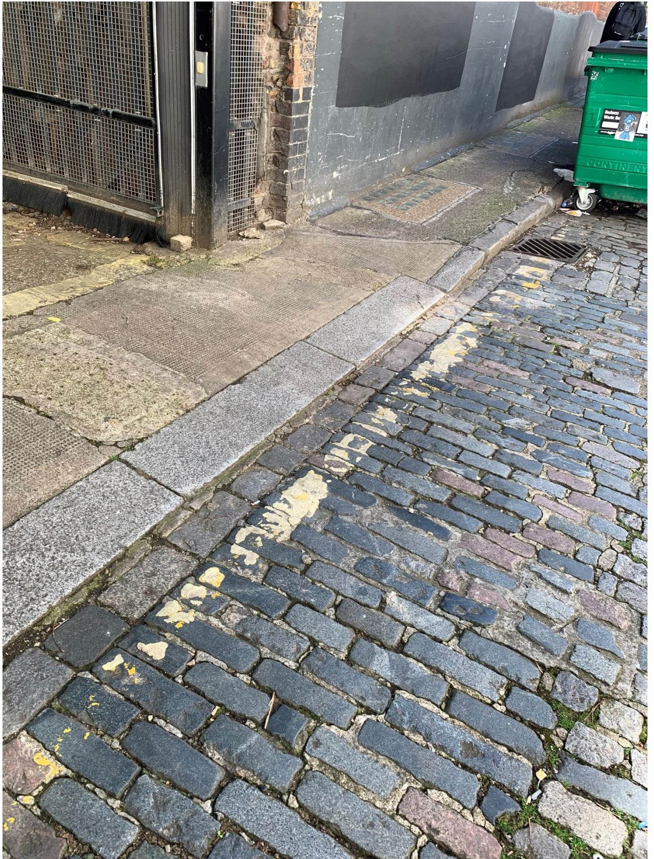
Photo 3: A detailed photo, showing the present condition of the granite setts and dropped granite kerb.
