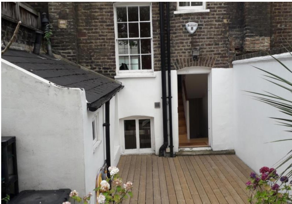
Fig 2. Photo of existing rear elevation.
