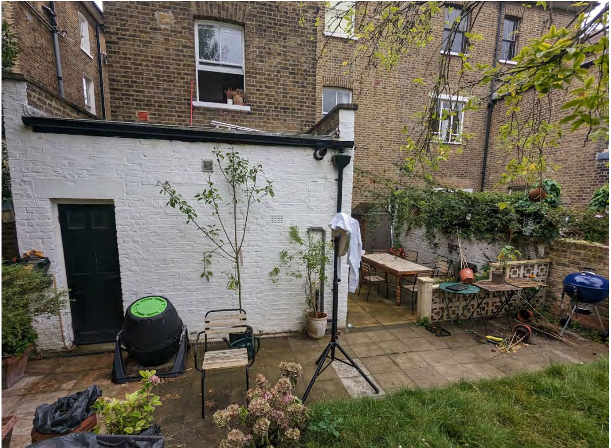
Photographic plate showing the existing rear elevation of the house.
