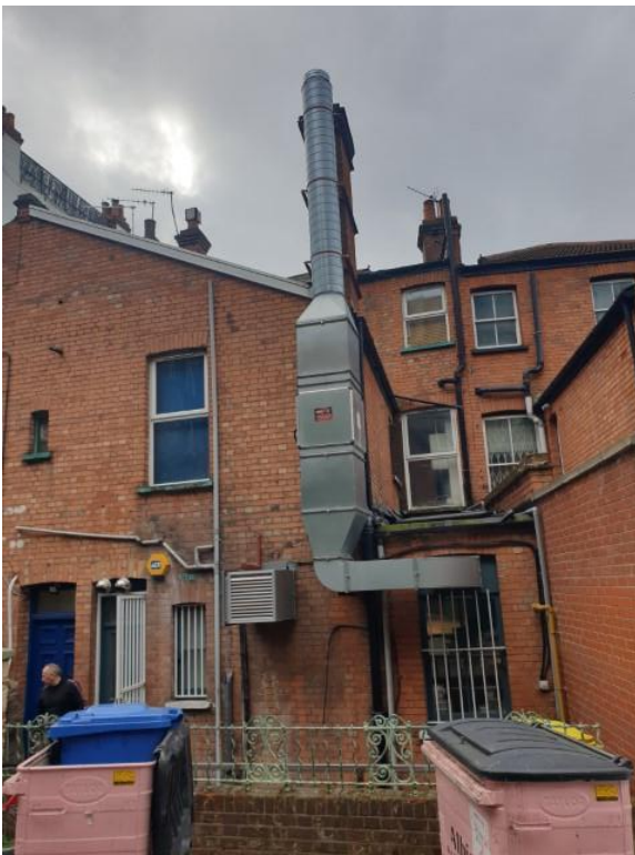
Figure 2: Rear of shop, existing flue runs up chimney
