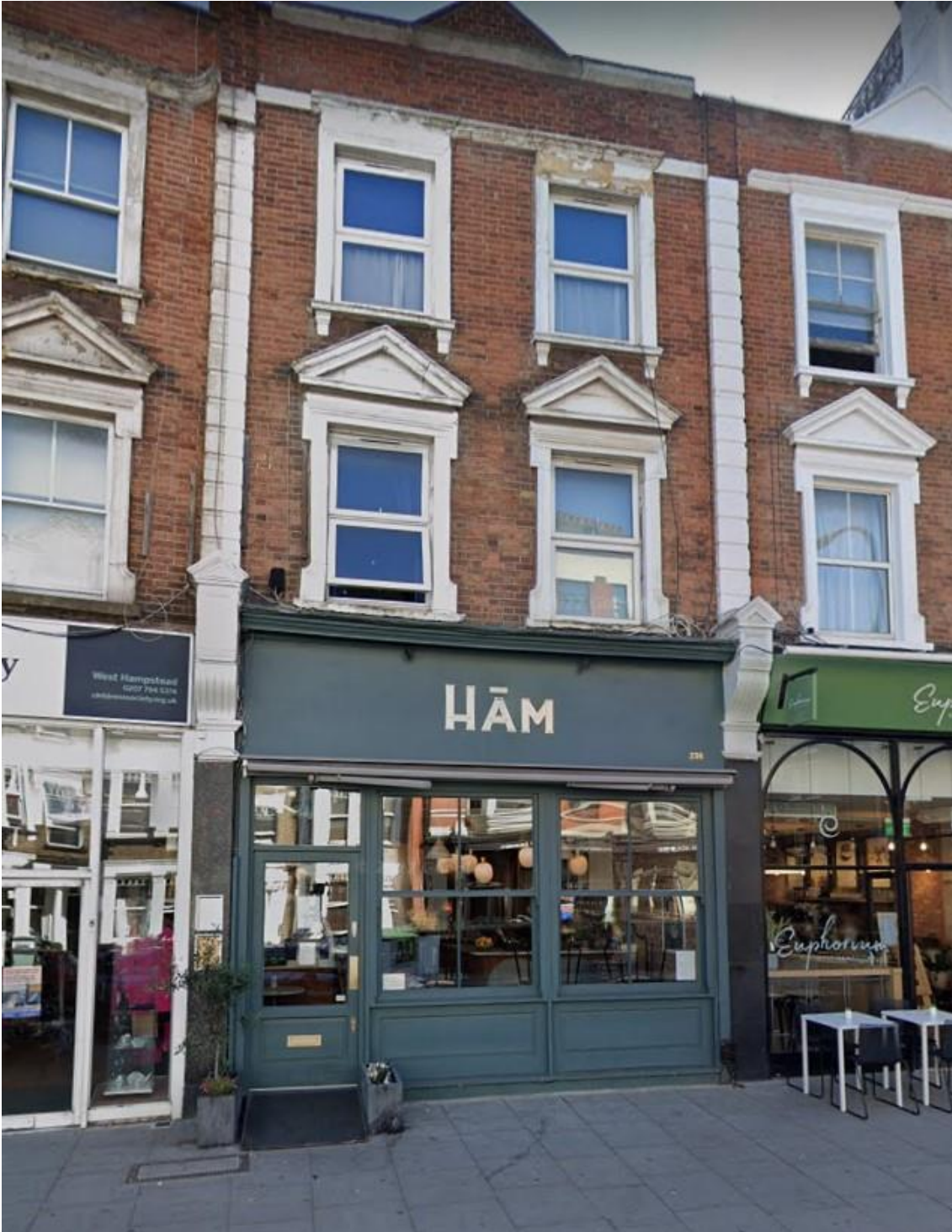
Figure 1: External view of the shop frontage.
