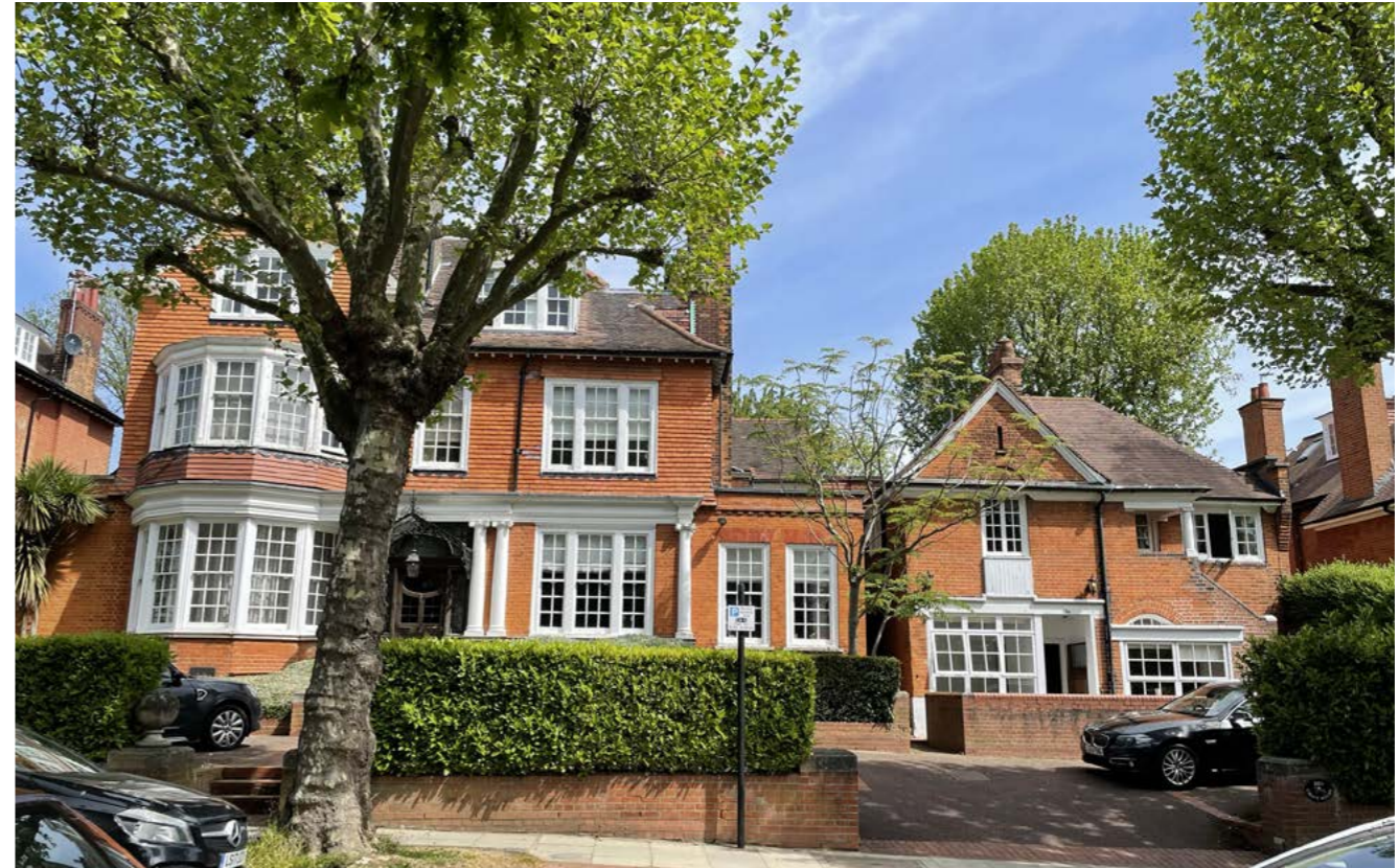
Fig. 8. Front view of 26A Ferncroft Avenue and neighbouring buildings
