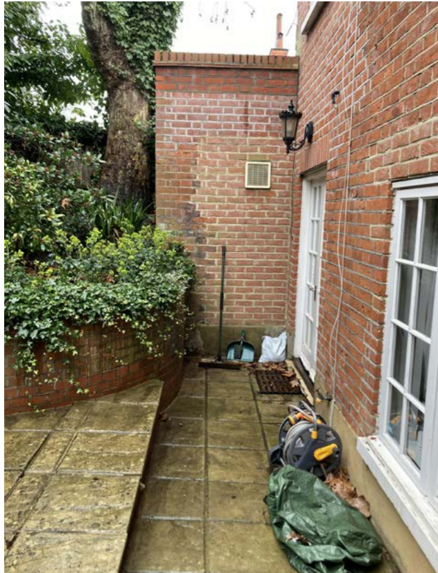
Fig. 57. Rear terrace looking south-east towards kitchen extension
