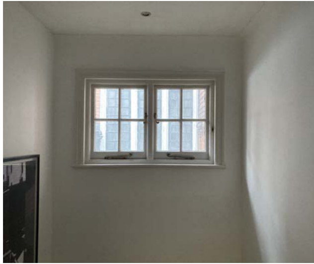
Fig. 41. Window at top of staircase, facing no. 26 Ferncroft Ave
