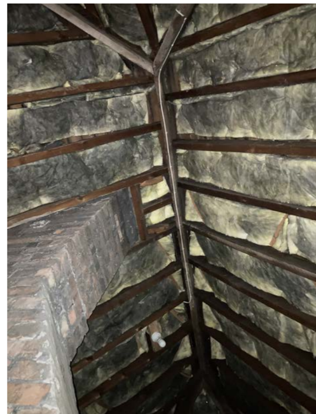
Fig. 55. Attic and brick chimney
