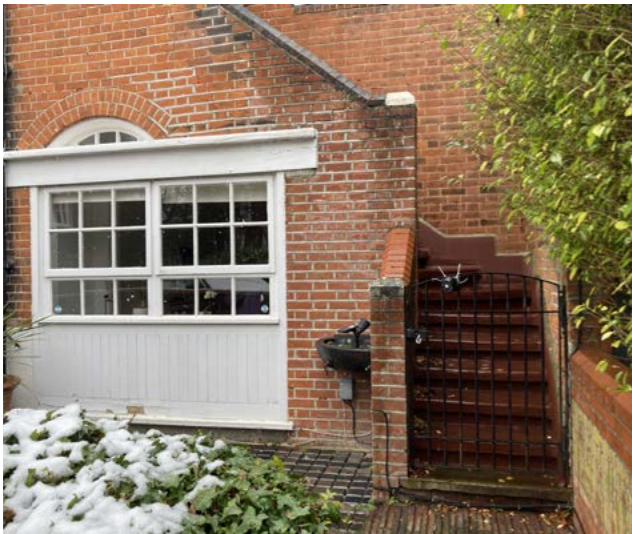
Fig. 26. External staircase to south east
