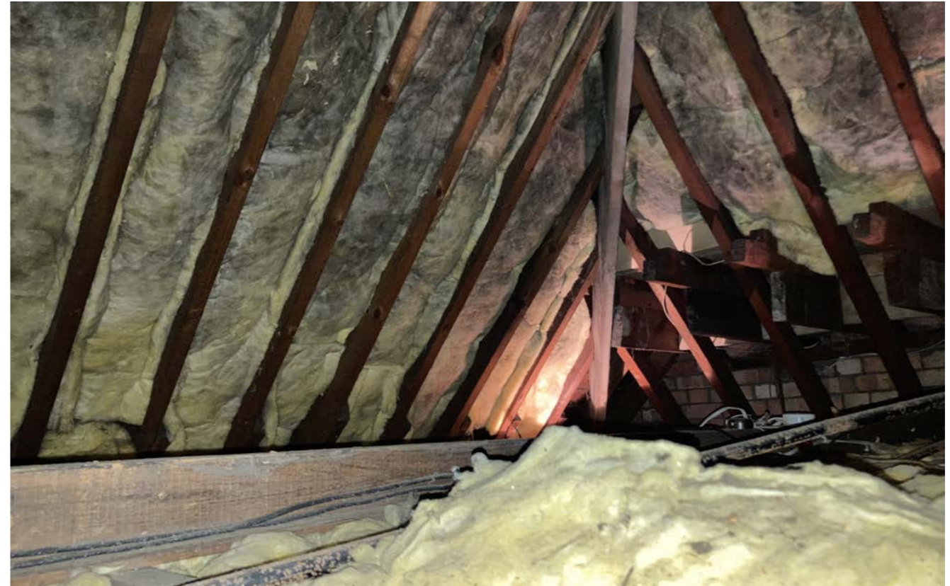
Fig. 54. Attic - light visible from 1st floor below
