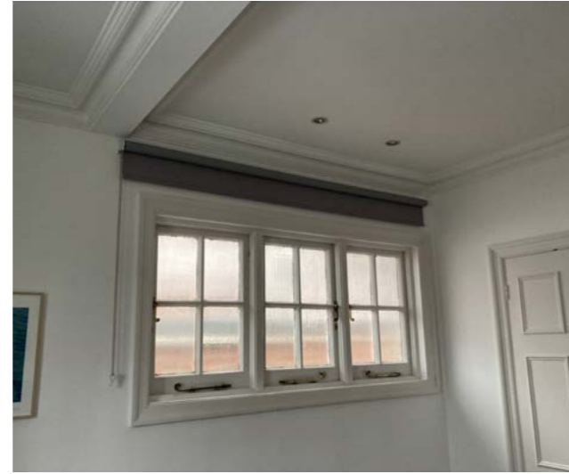
Fig. 44. Window in 1st floor study, facing no. 26 Ferncroft Ave
