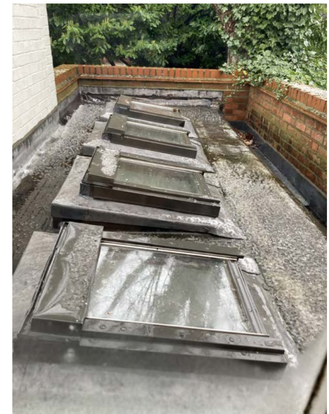
Fig. 49. Rooflight above kitchen window
