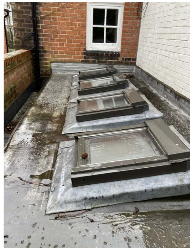
Fig. 60. Roof and rooflights to kitchen extension
