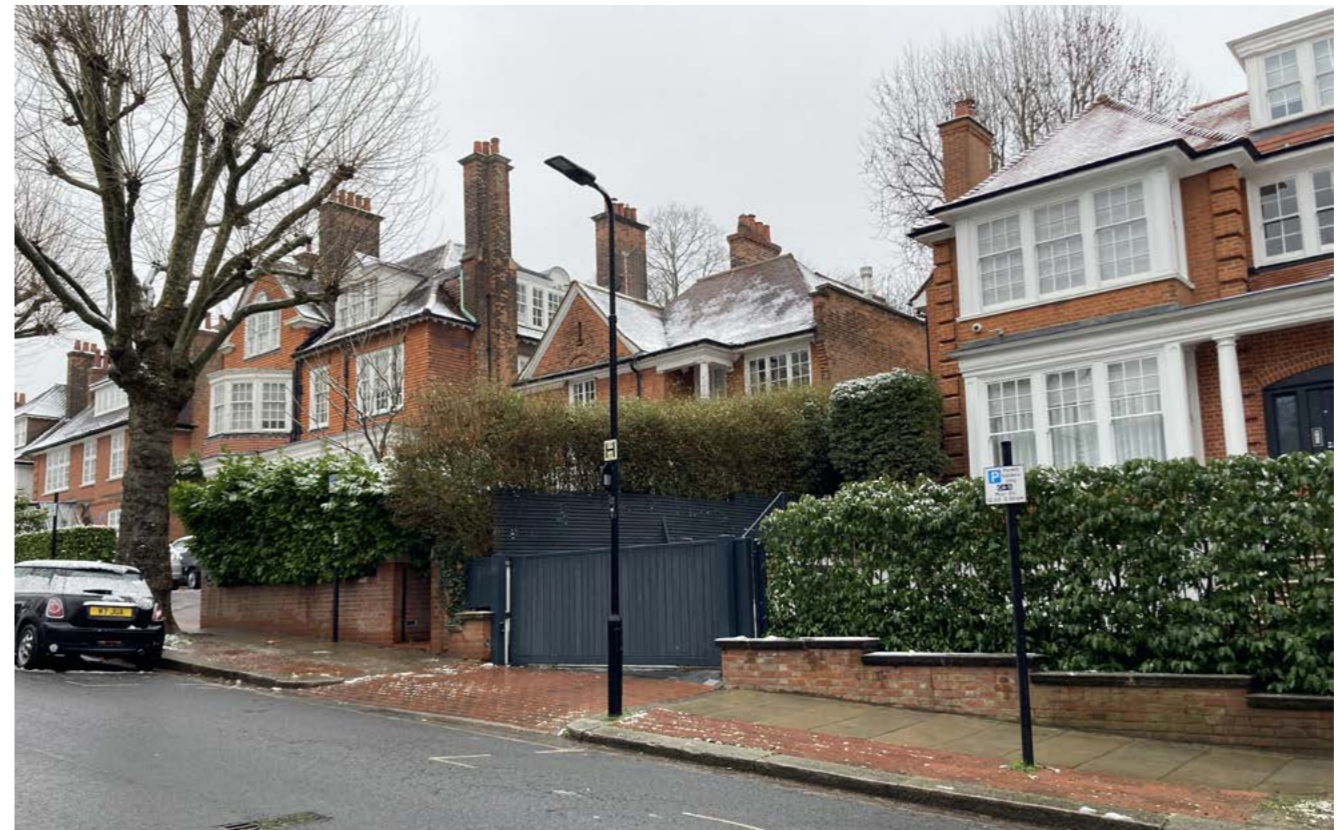
Fig. 9. Front view of no.26 (left) to 28 Ferncroft Avenue (right)
