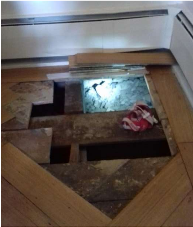
Main living room parquet floor, showing thin timber veneer strips applied to backing floorboards (which are of no significance)
