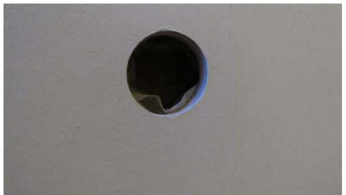
This removed downlight in the utility confirms the ceiling is modern plasterboard
