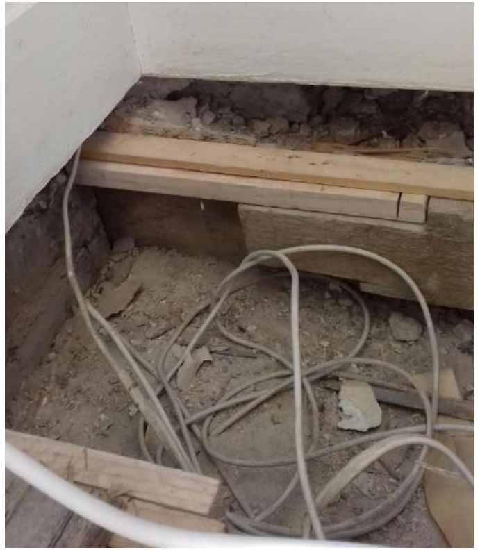
Master bedroom floor, showing severely notched historic floor joists
