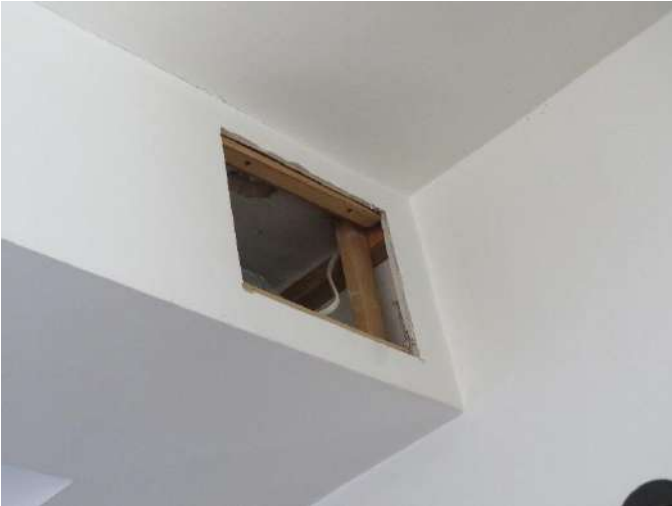
This opening in the ceiling boxing in the kitchen shows that this is entirely modern and accommodates modern services only
