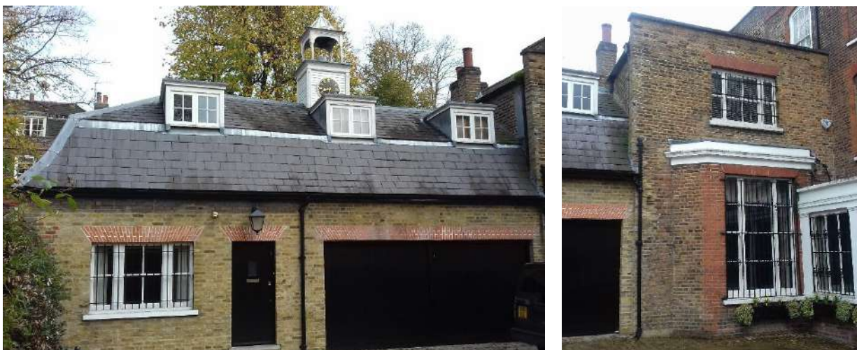
Figure 39: 19th-century side extension with modern alterations to the garage door openings and surrounding brickwork. The old courtroom (now billiards room) is shown on the right
