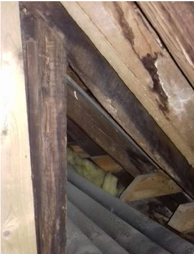
Hatch opened to view roof eaves - modern timber rafters and services.
