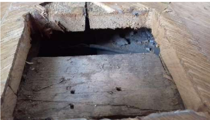
This is the opening from a removed floor grill in the floor in the lounge (within the 19th-century extension). The parquet is exceptionally thin, applied modern floorboards. The joists are historic.
