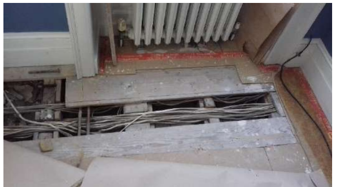
The floor of the master bedroom, showing historic (but not original) and historic joists, which are severely notched to facilitate modern services.
