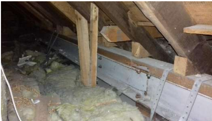
Hatch opened to view roof eaves. Modern steel beam and many modern timber rafters, evidencing modern replacement of roof
