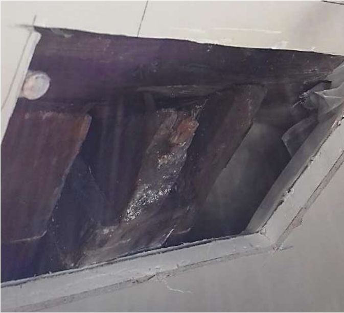
Opening next to roof light shows a mix of timber rafters, suggesting some reuse of old timbers in modern replacement roof
