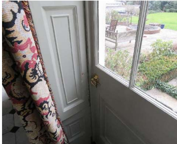
Figure 29: Original moulded timber shutters
