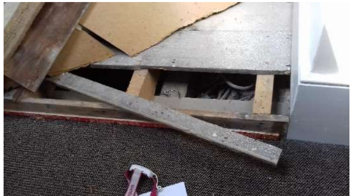
Raised floor 2 nd -floor studio space – modern, to accommodate services.
