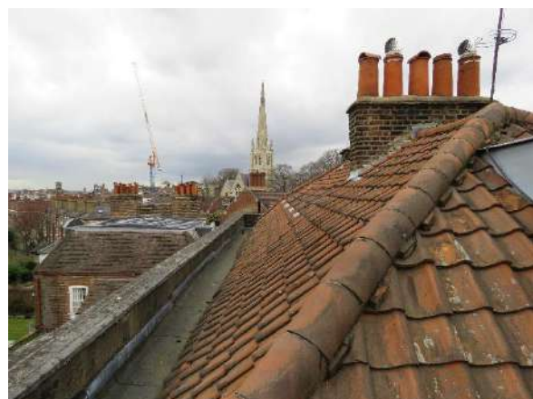
Figure 35: Roof with modern pantiles
