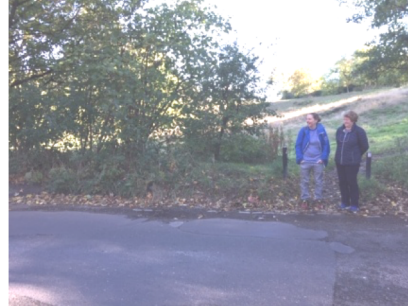
3. Branch Hill by culvert
