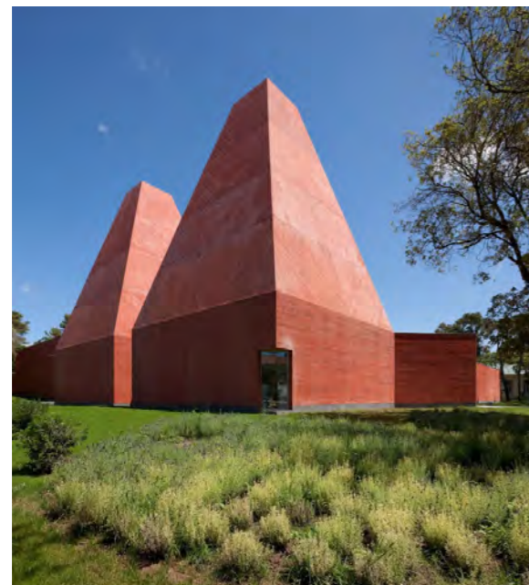
4. Concrete roof form by Eduardo Souto de Moura
