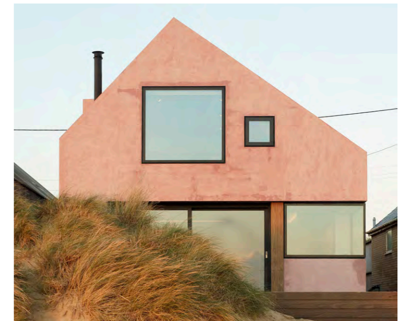
7. Pale red concrete finish trowel applied at Seabreeze, West Sussex by RX Architects
