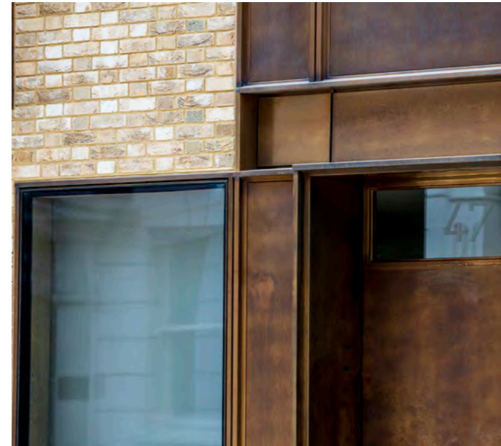
2. Old Church Street bronze framed and minimal framing window fenestration
