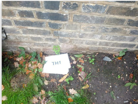
Fig 1.1: Trial Hole 1 Location
