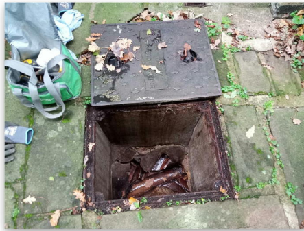
Fig 3.1: Defective manhole
