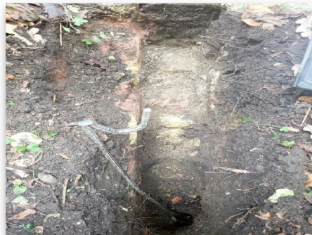
Fig 2.2: Trial Hole 2 Footing
