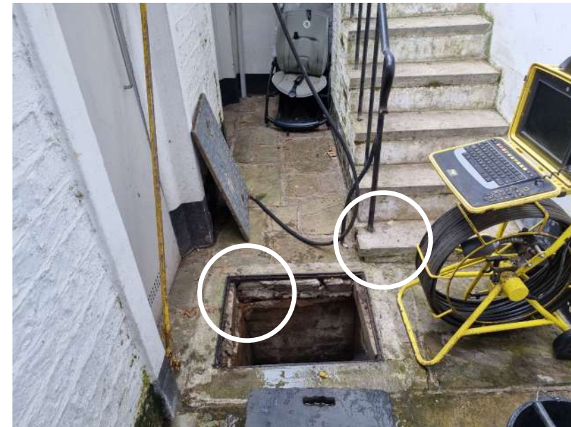
Figure 4: Lightwell to Street Staircase. The first step is also shorter than subsequent steps here. The buildup on top of the original floor can also be appreciated from inside the manhole.
