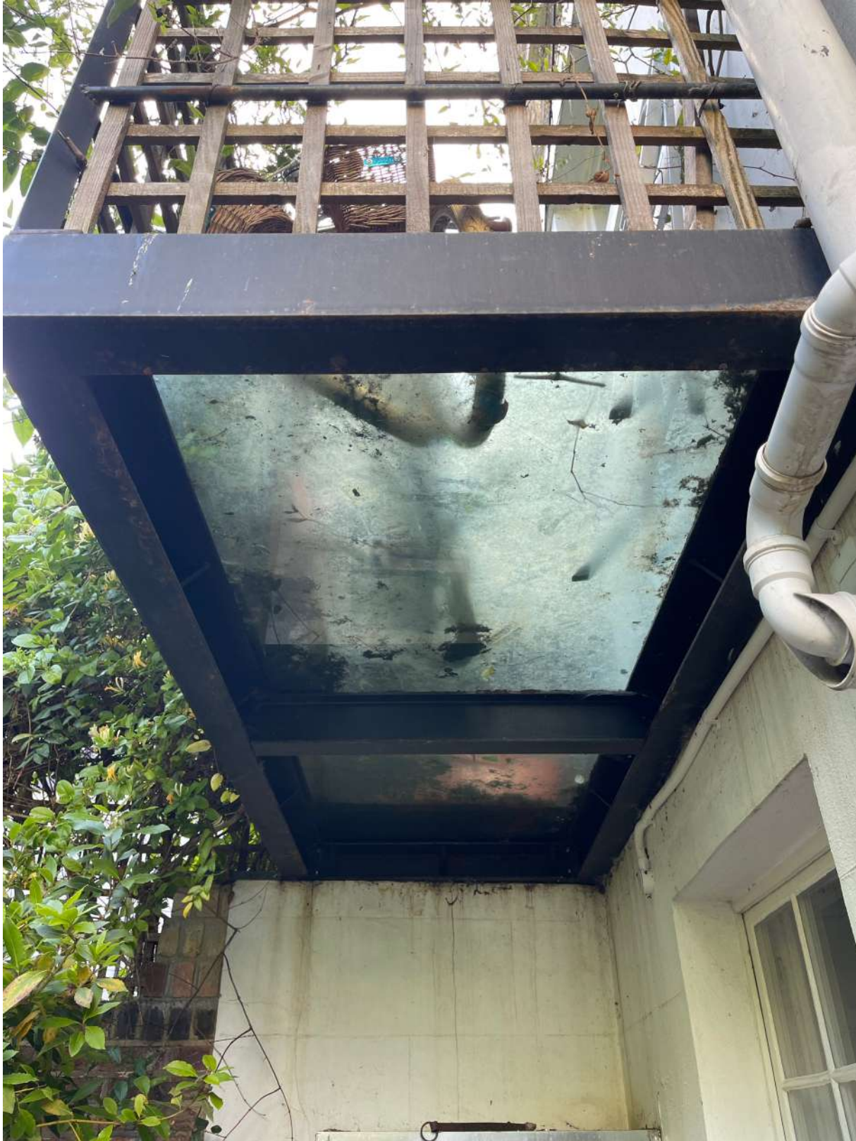
Figure 7: Materiality of existing ground floor balcony. Metal and glass.
