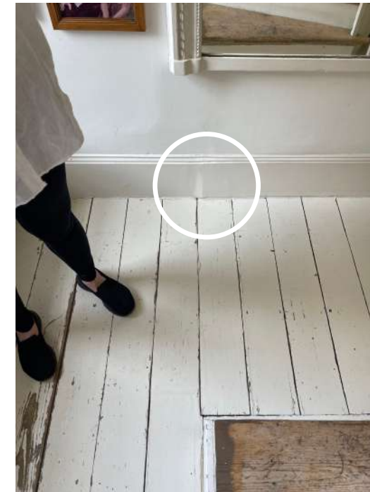
Figure 8: Break in skirting in First Floor hallway opposite staircase suggests this might be the line of the original wall before it was removed. The proposal seeks to reinstate this wall in order to create a vestibule.
