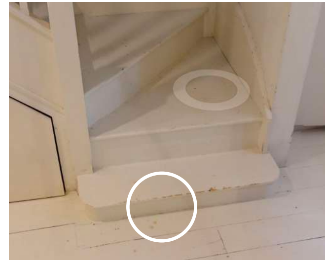
Figure 3: Lower Ground to Ground Staircase. First step is considerably shorter than subsequent steps suggesting that the level of the Lower Ground Floor is currently too high compared to original.
