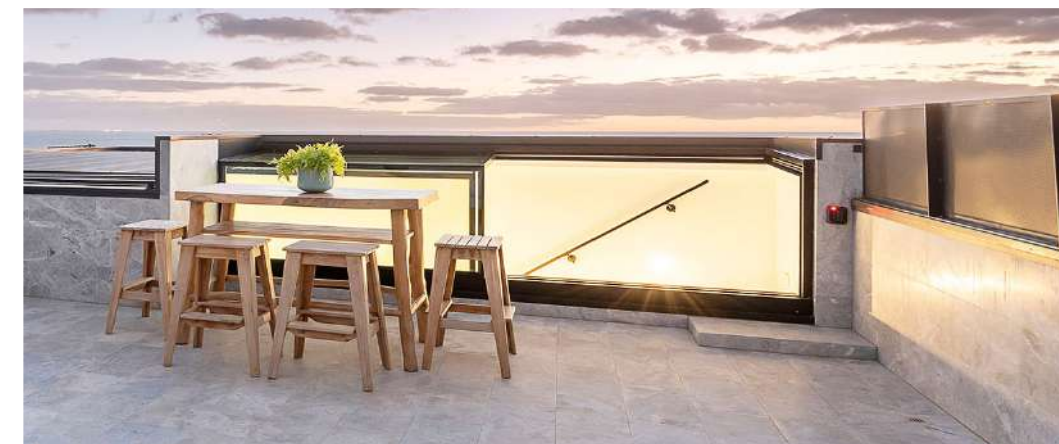
Figure 10: Example image of roof access box below the level of the parapet. The proposal will also have a section of the roof box which slides over the other half in order to create opening and provide the headroom required to accommodate staircase.
