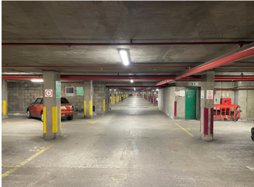
GENERAL LONG VIEW OF THE CAR PARK
