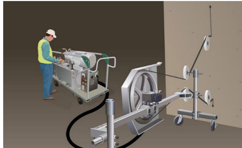
Diamond Saw Cut
