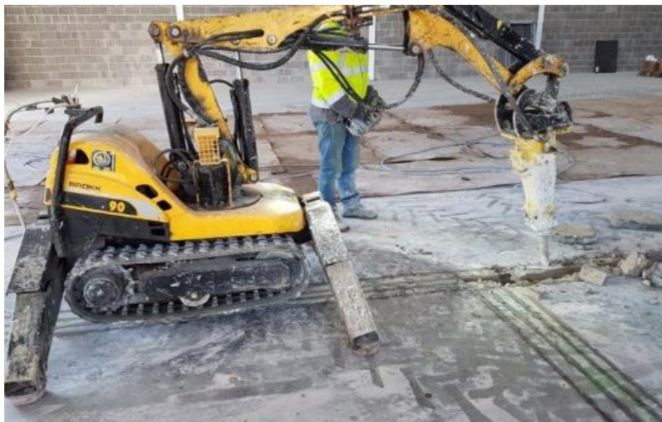
Jacking and Slab Cut Out
