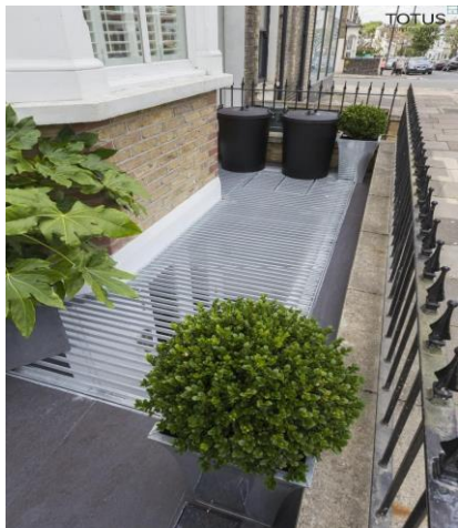
Sample photo of lightwell from Totus construction at Clapham
