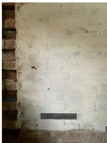
No 1: One-part Pozzolan Limewash one-part water.
