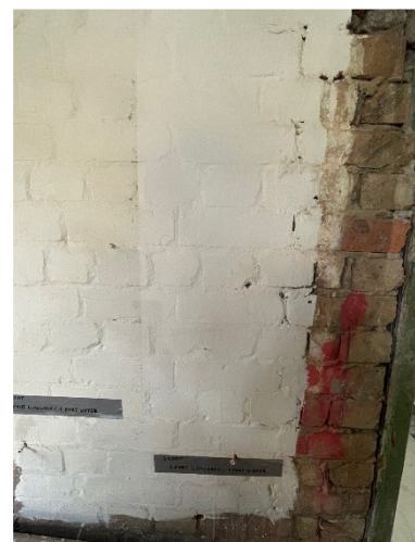
No 3: One-part Pozzolan Limewash one-part water plus two coats exterior limewash
