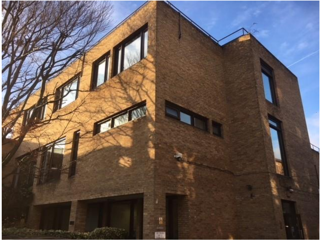
Photo 5- Rear/East Facing Elevation
