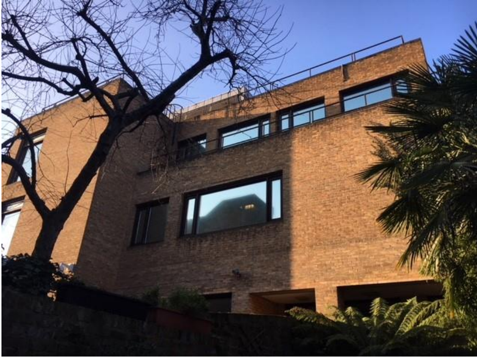
Photo 7- East Facing Elevation
