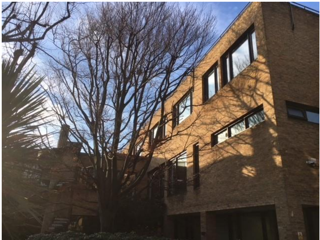
Photo 6- East Facing Elevation
