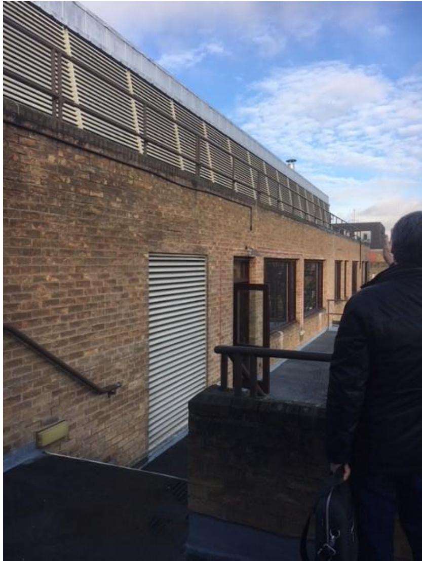
Photo 3- Looking East from Third Floor
