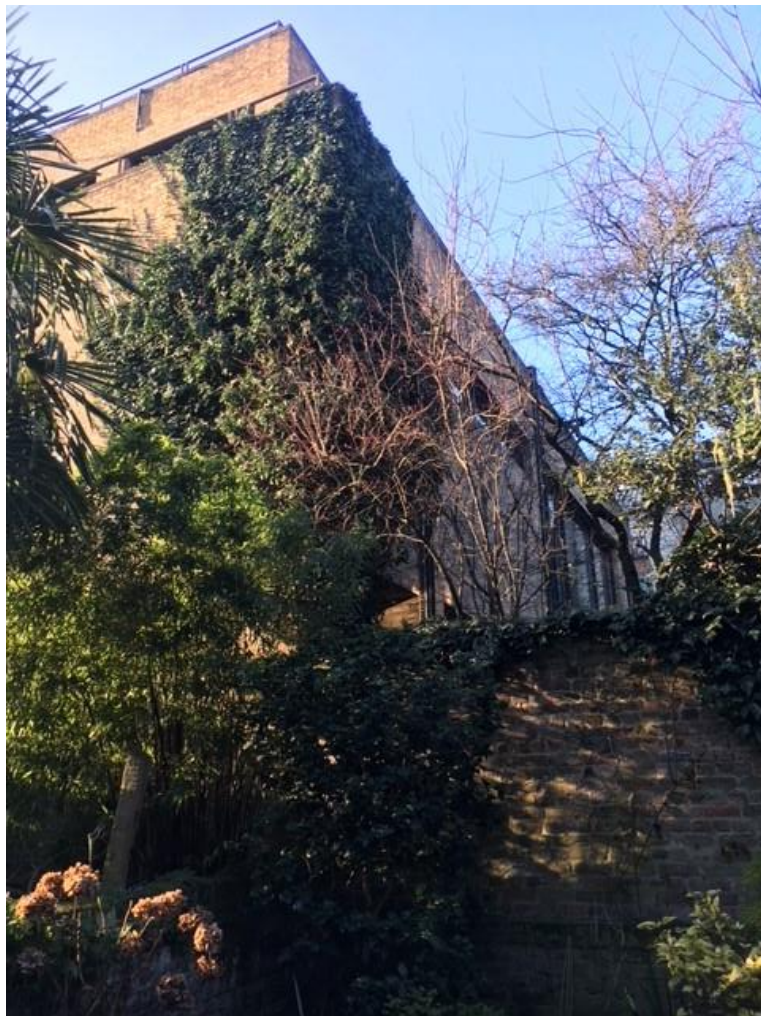
Photo 8 – North Facing Elevation
