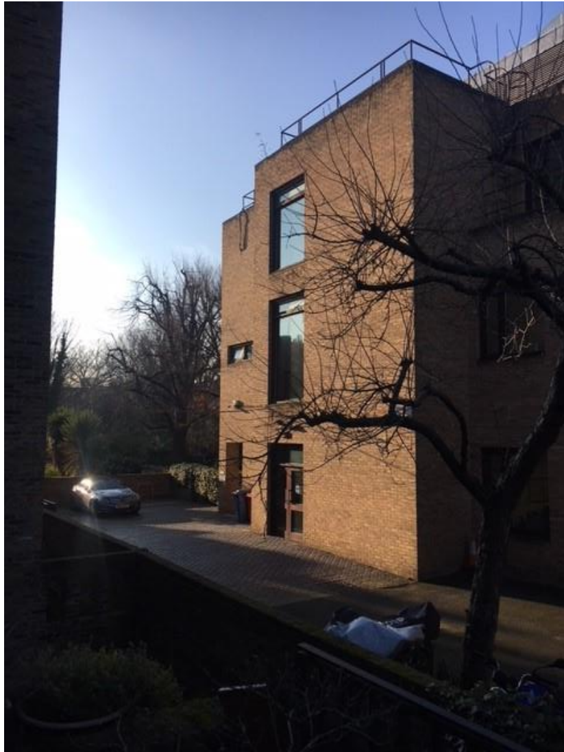
Photo 9- East Facing Elevation
