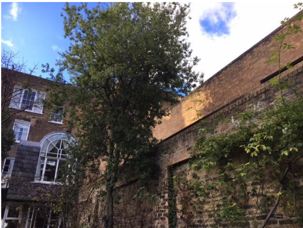
Photo 11-View of Rear Elevation of 118 Albert Street and Shared Boundary Wall
