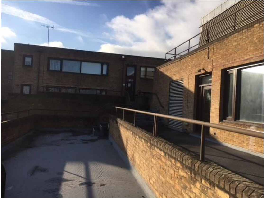
Photo 2- Looking West from Second Floor Roof
