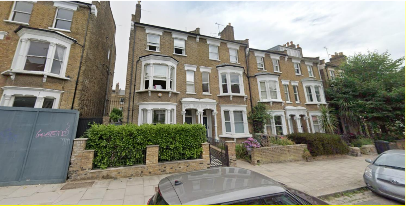
Photo 3 (above): Street view photograph (source:Google 3D)
