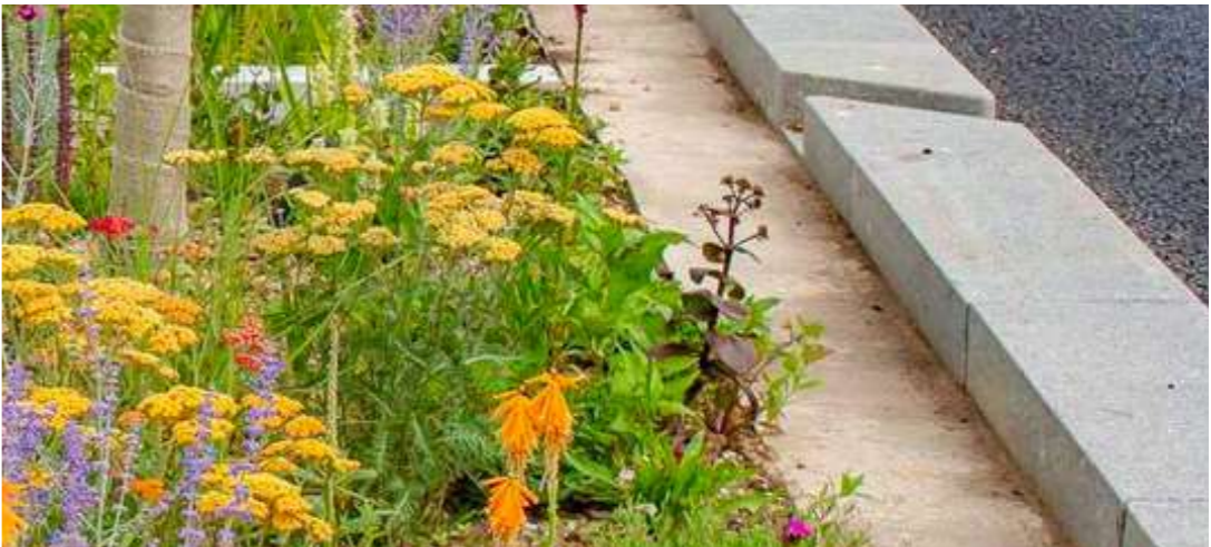
Rain garden planting with surface drainage slots
