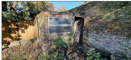
Picture showing the existing Boundary Wall Between 14 GG and number 6CG.
