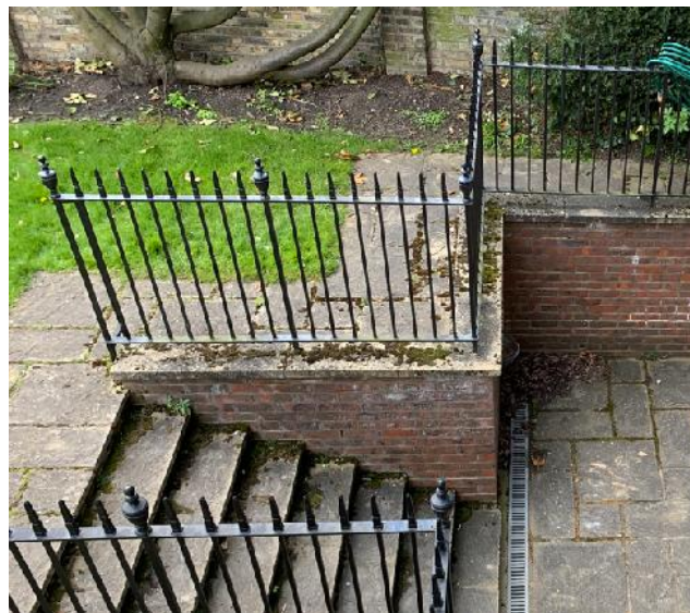
Further evidence of metal work as existing
