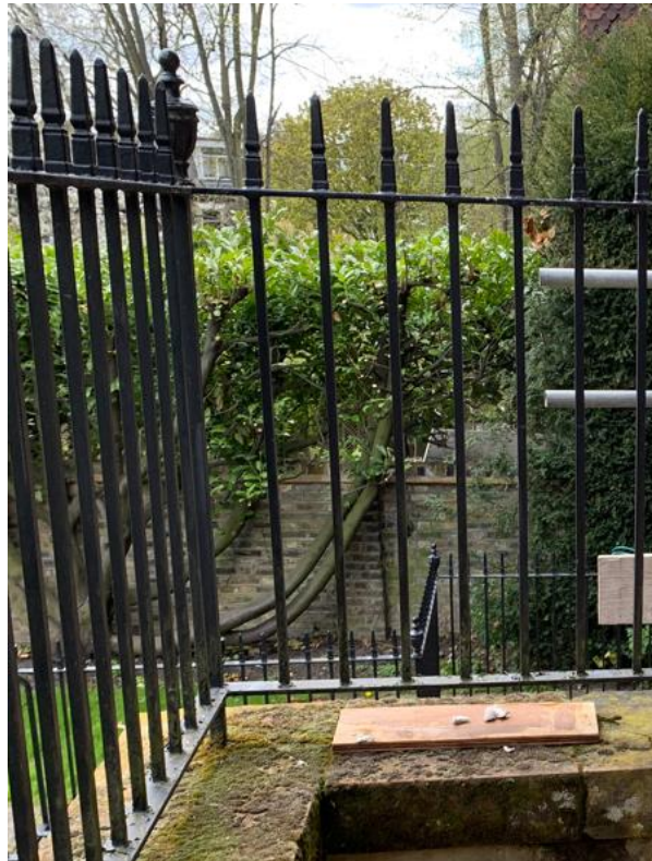
Existing metal work to rear terrace
