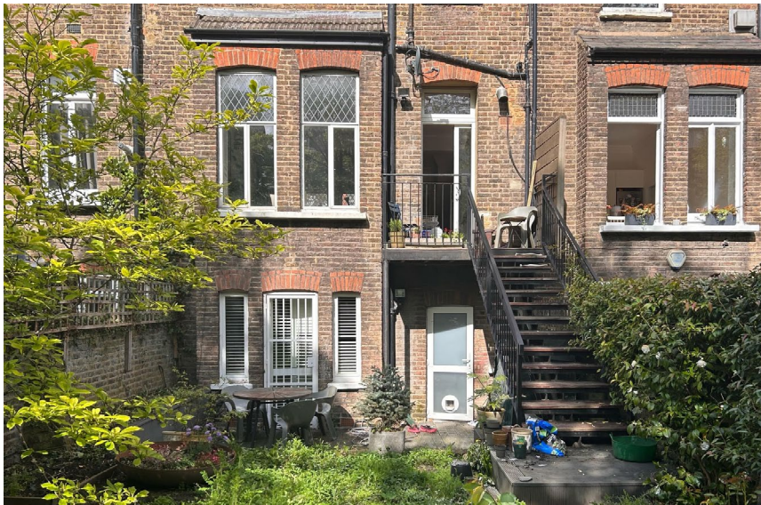
Figure 01 - Photo of rear elevation of 13A Primrose Gardens
