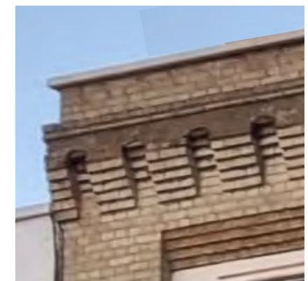
Feature masonry details at coping
