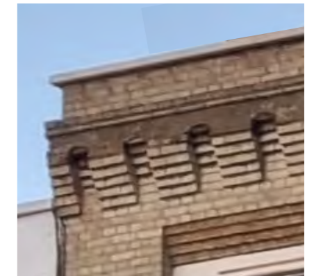
Feature masonry details at coping
