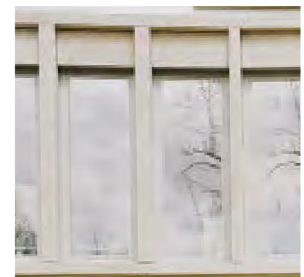
Stone surround to windows
