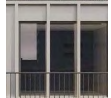
Wet-cast stone fins and spandrel to pavilion
