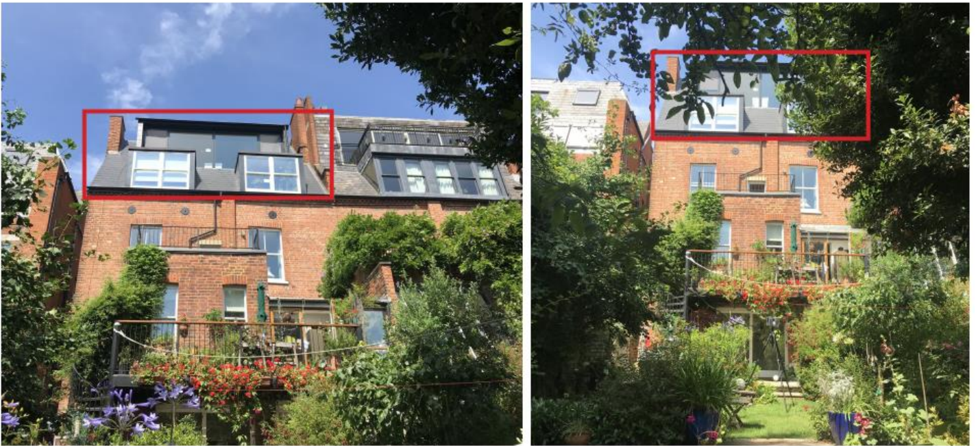
Fig.1. Photos of Rear Elevation
