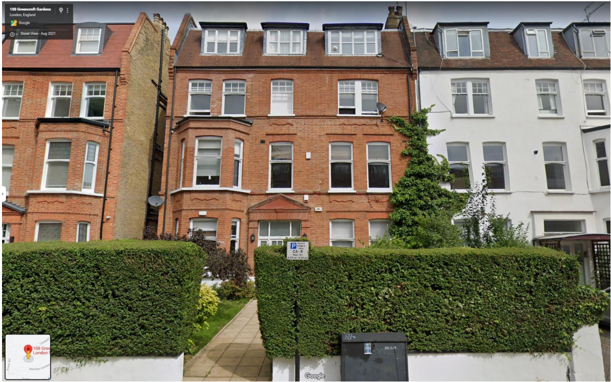
Photo 4: Front elevation, host property from street.
