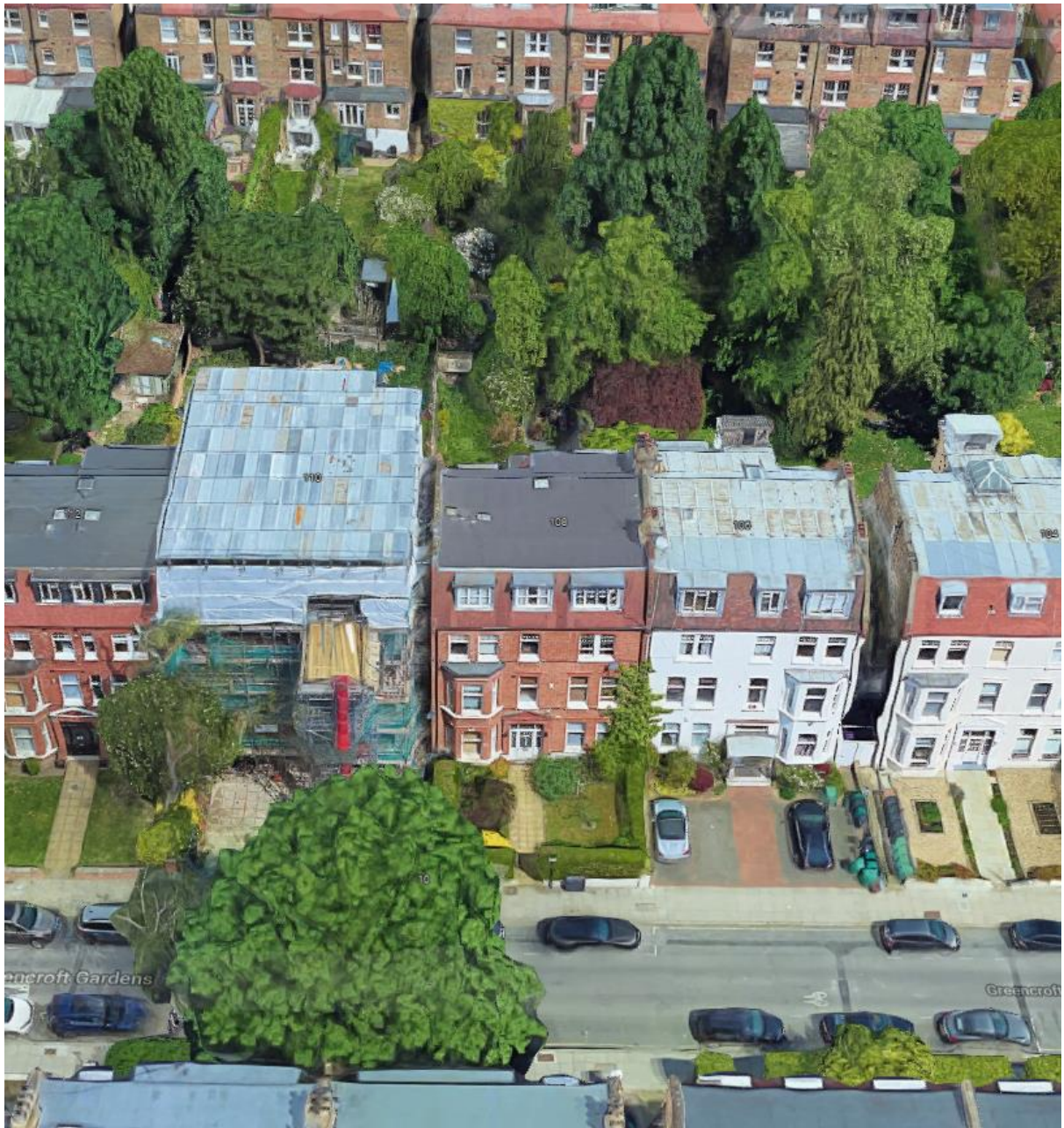
Photo 1: Aerial view facing front elevation. (Neighbour, no. 110 with scaffolding.)
