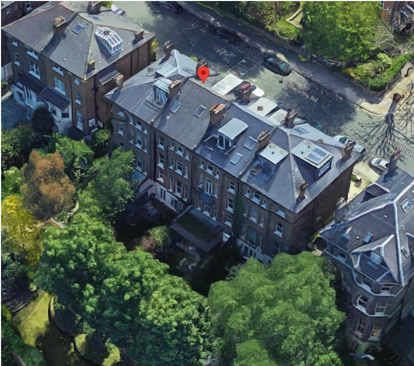
1. Aerial view of the rear elevations showing variation of lower ground floors within the terrace
