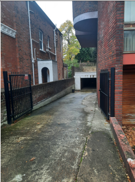
Fig. 2. View between Nos. 8a and 10 Hampstead Hill Gardens
