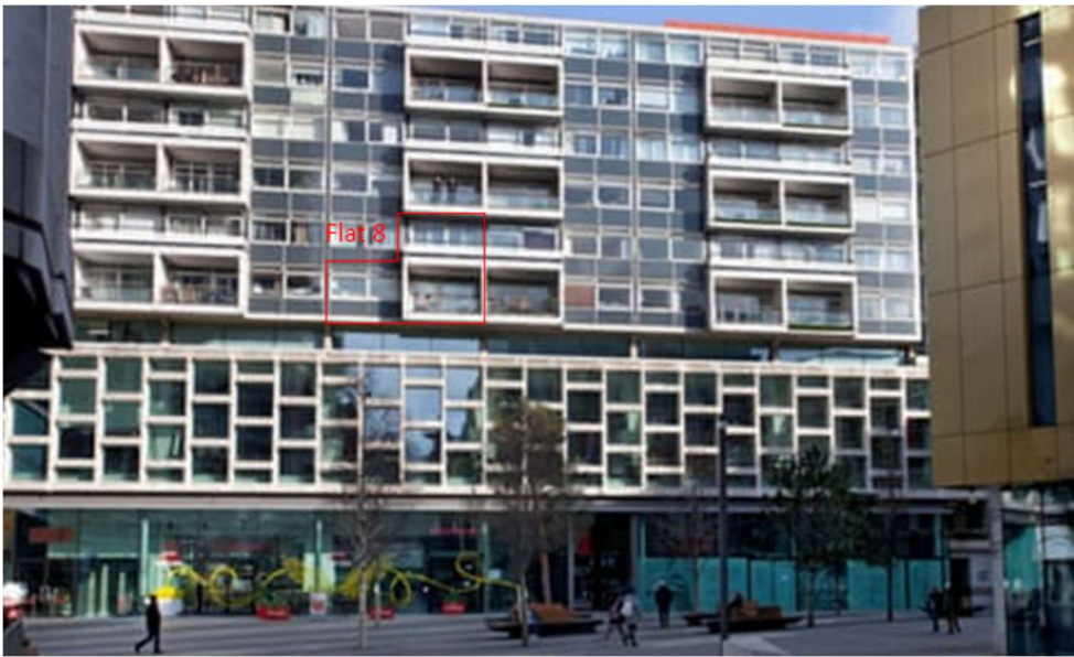
Centre Point House, West Elevation, view from below Centre Point. (Flat 8 elevation outlined in red)
