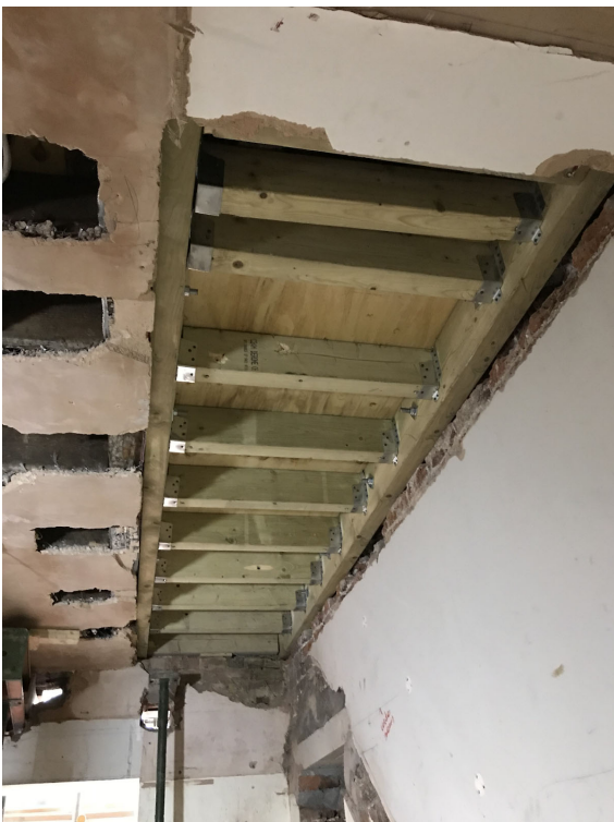
Exposed timber joists in 2018. Modern timber joists of the new floor can be seen.
