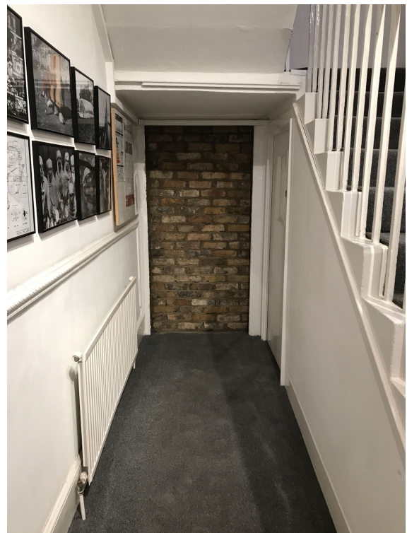
New brickwork blocking openings to rear elevation made in 2018.
