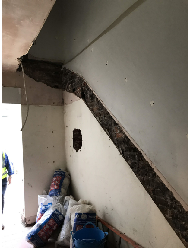
Removal of staircase down into the basement in 2018.
