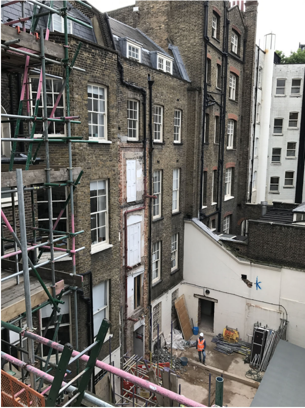
Removal of the toilets at no.38 and internal doors revealed in 2018.
