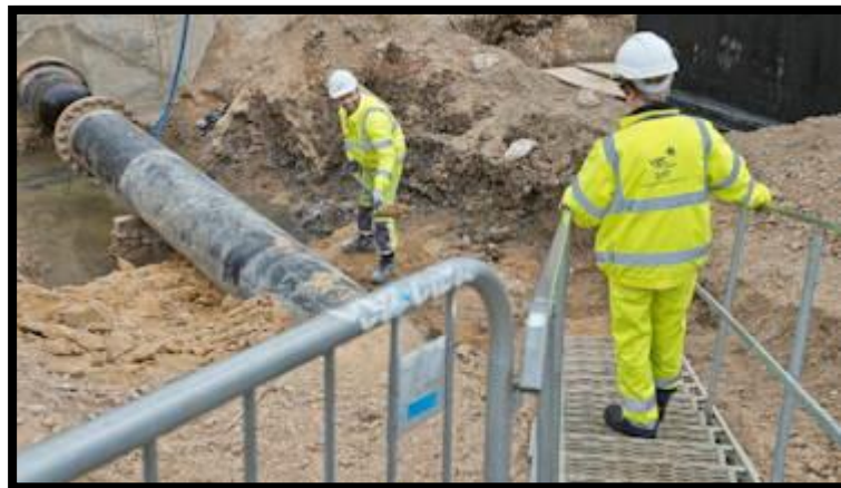
Figure 19 Safe access to excavated area
