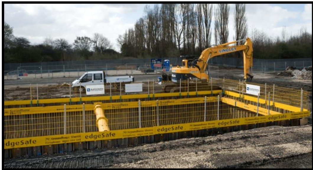
Figure 18 Edge protection for excavated area by edge safe
