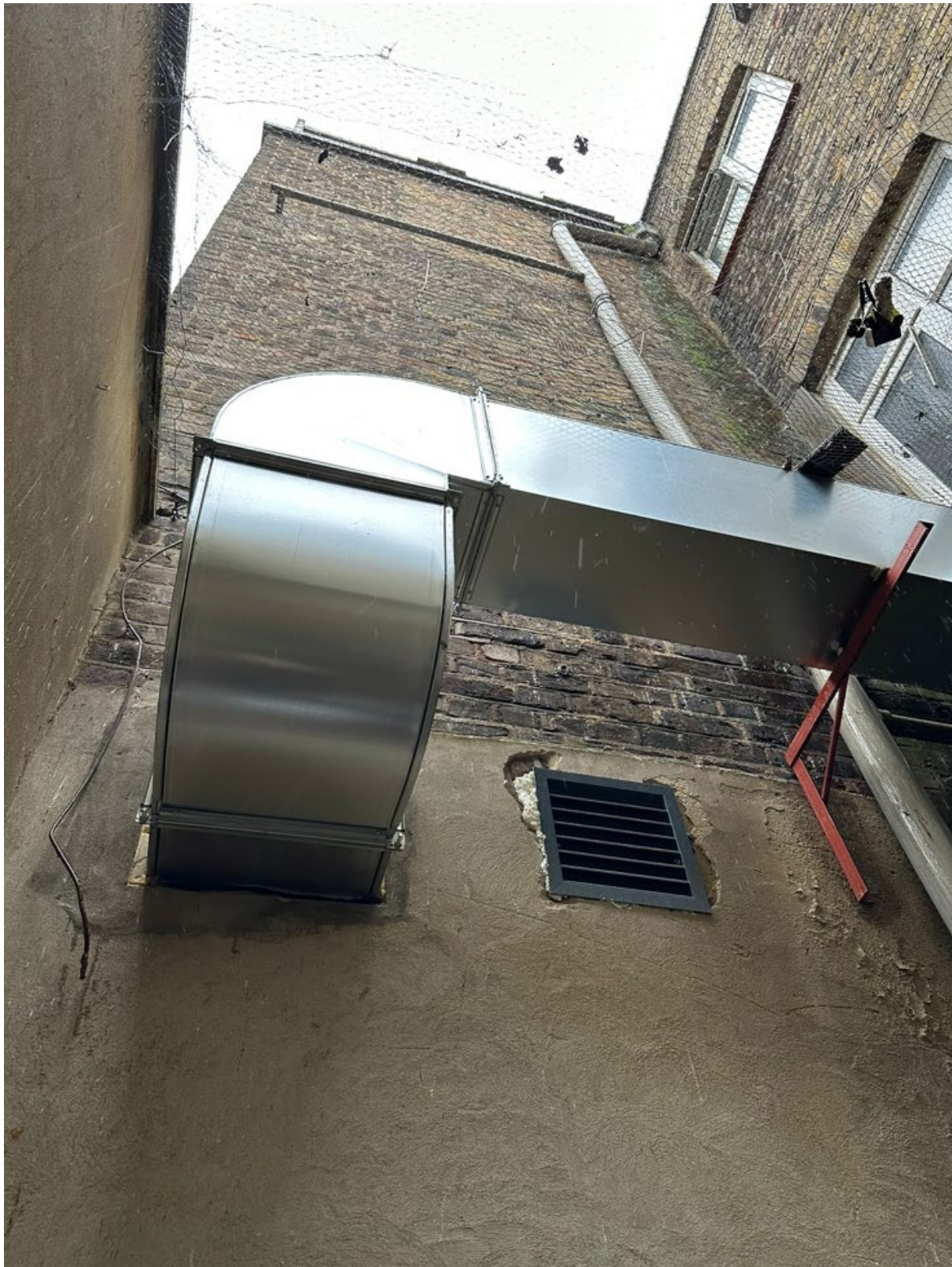
Photo 2 View of exhaust ductwork penetrating the facade
