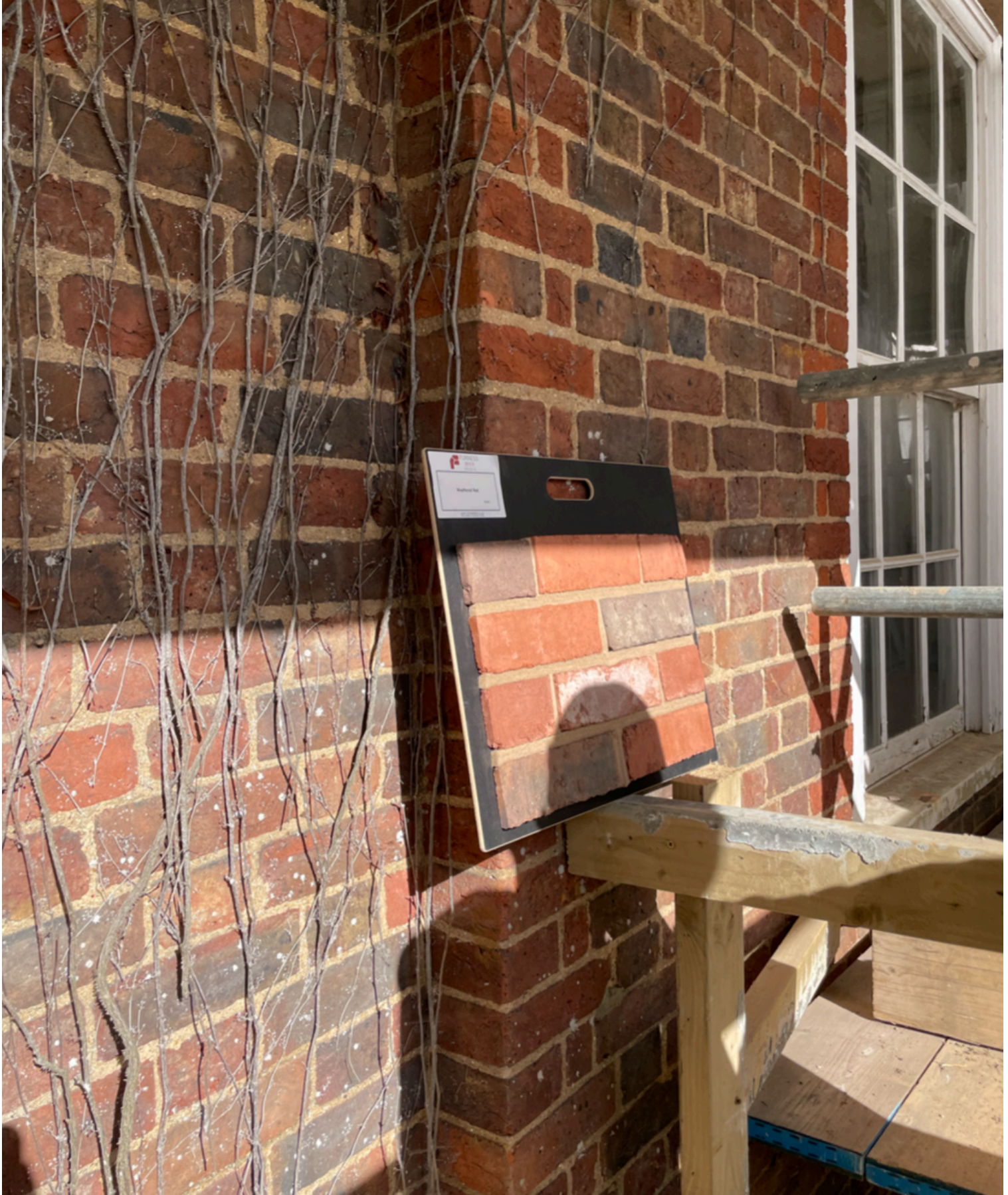
Material 01 New facing brickwork to basement extension Furness Brick & Tile Co Ltd Clamp Range - Weathered Red with Natural Orange detail Cement lime mortar mix to match existing
