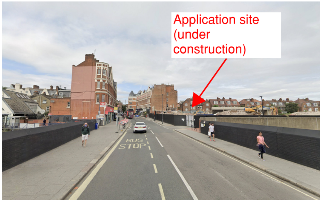
Image 1 – looking north along West End Lane towards application site
