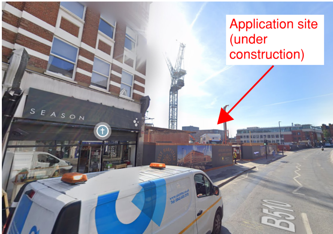
Image 2 – looking south along West End Lane towards application site
