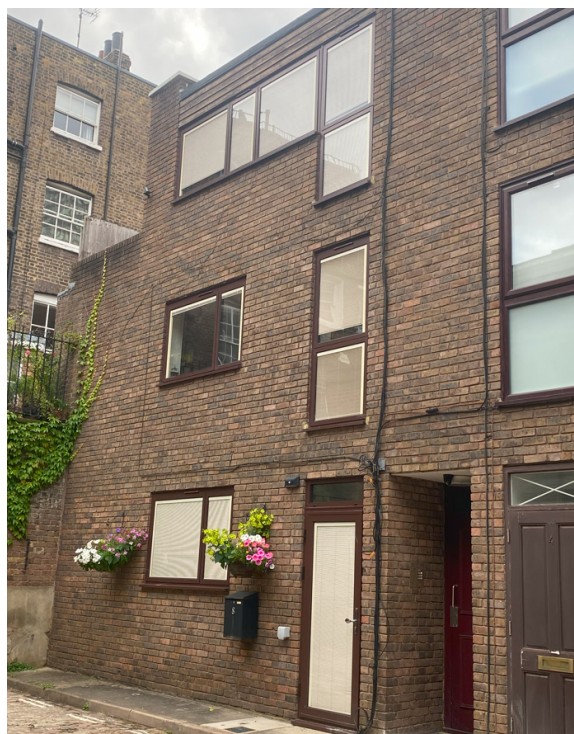
Image 6 – showing integrated blinds to south-facing windows as part of solar shading measures taken
