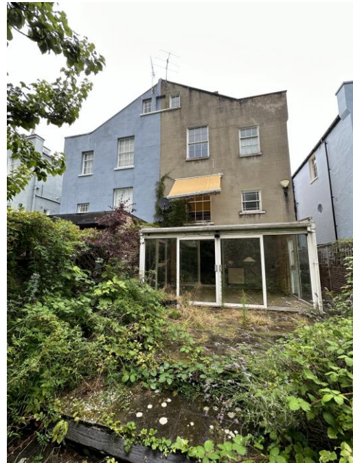
Figure 13 The rear façade of the building.
