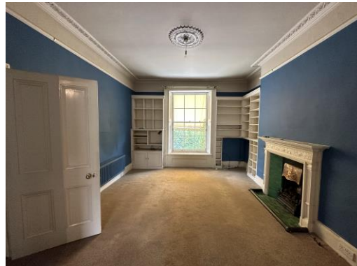
Figures 18 & 19 The front room (top) and rear room (bottom) at ground floor level.
