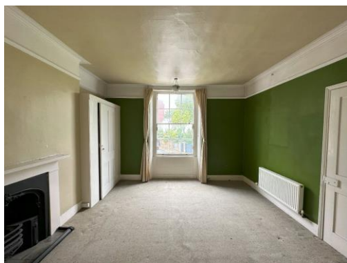
Figures 20 & 21 The front (top) and rear (bottom) main rooms at 1 st floor level.
