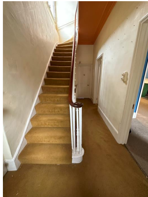
Figure 14 The main ground to 1 st floor staircase.
