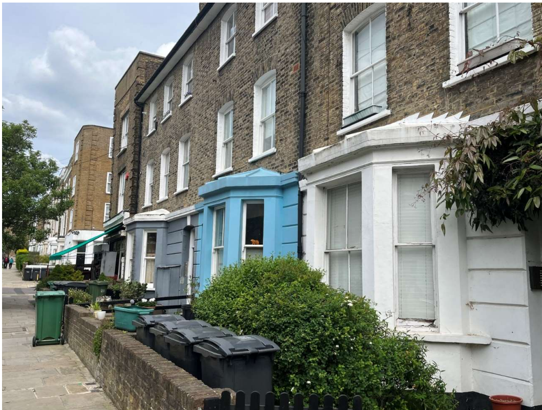
Figure 9 Photo showing the alignment of the front of the new storage unit to the adjacent bay windows.
