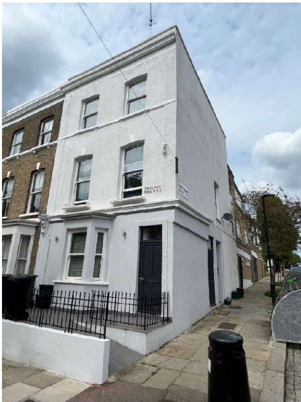
Figure 21 - Falkland Store, 71 Falkland Road NW5 2XB: Was unoccupied for 2 years. LPA gave permission to be converted into a dwelling unit in February 2017 (2016/1562/P).
