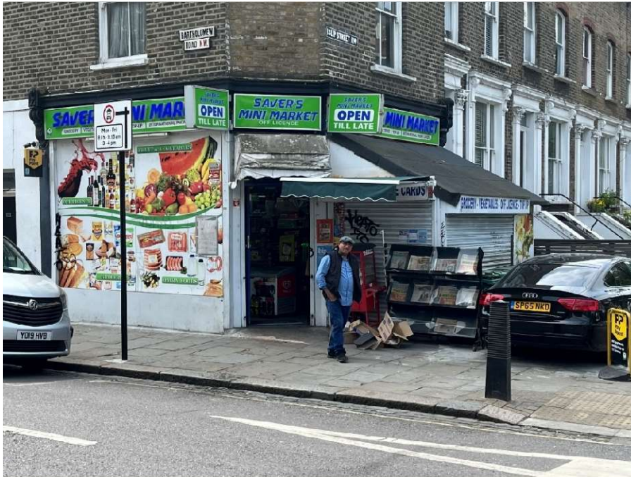
Figure 22 Saver's Mini Market, 121A Islip Street NW5 2DL: Had to extend out onto shop forecourt with full openable enclosure
