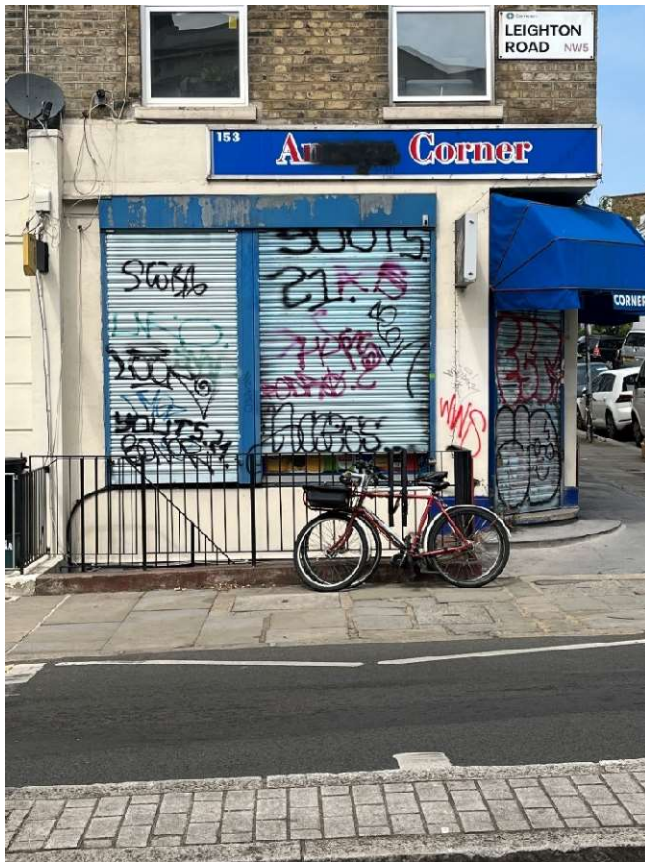
Figure 19 - Susan's Mini Market 153 Leighton Road NW5 2RB: (now renamed as Amaya Corner) hasn't created any new storage and appears to ceased trading leaving, it is in a state of neglect.
