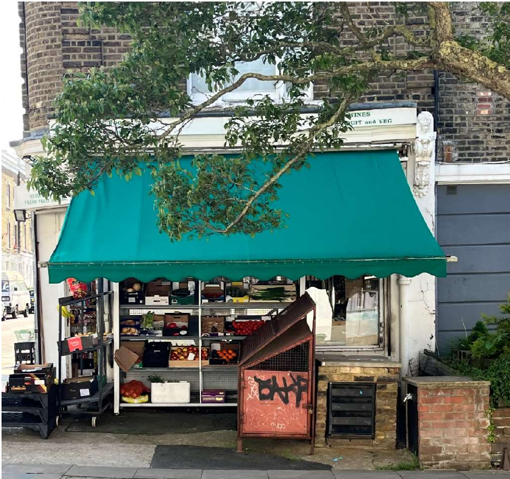
Figure 10 Photo showing visibility of the new storage unit when shop is open.
